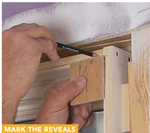
MARK THE REVEALS
