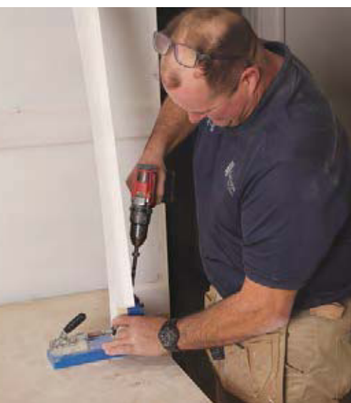
SCREWS JOIN STOOL SEGMENTS
