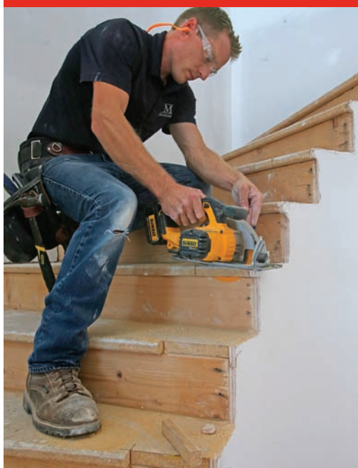
Prep the rough stairs. Radius-edged rough treads are cut flush to the rough risers to create an accurate reference point for measurements and to clear the way for the false tread caps that come later.
