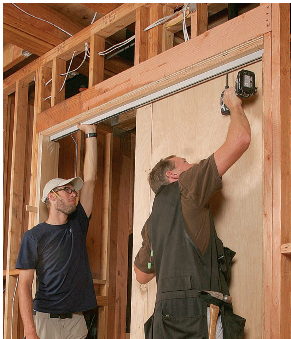
Install the track. Fasten the track to two layers of \frac{3}{4} -in. plywood attached to the bottom of the structural header. The plywood provides a straight, twist-resistant surface and bridges the gap that's in the center of a two-ply header, which is where the track-mounting screws go.
