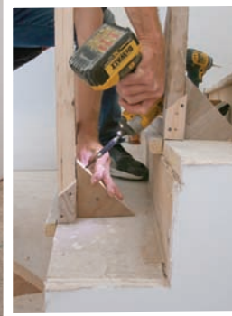
Bending brackets. Fastened 6 in. from the open end of each tread and parallel to the face of the risers, site-made brackets become the handrail bending form. The brackets at the upper and lower ends of the stairs are also braced laterally (inset) to resist the forces of the rail as it's pushed against the form.
