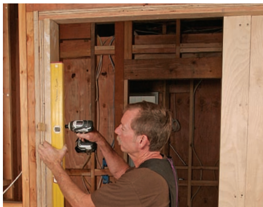
Fasten the strike jamb. Using opposing shims, plumb the strike-side jamb, and fasten it every 8 in. with pairs of trim-head screws. A 6-ft. level ensures that the jamb is straight throughout its length so that it will make full contact with the edge of the door.
