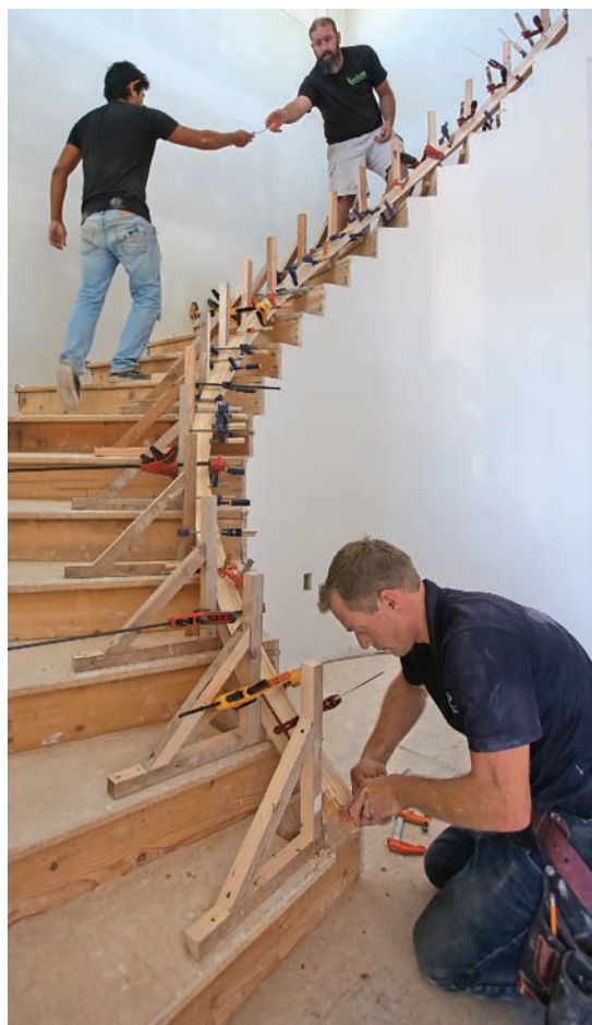
Aim for a fair curve. After its laminations are coated with wood glue, the poplar handrail is sandwiched together, held with a few bands of shrink wrap, and pressed into place against the form. When the rail is properly positioned, it should be tight to the face of each bracket, set down against the angled stops on each bracket that match the slope of the stairs, and twisted so that the bottom face is flat to the top of the treads. Holding the rail tight to all these critical areas requires a lot of clamps, so have plenty on hand.
