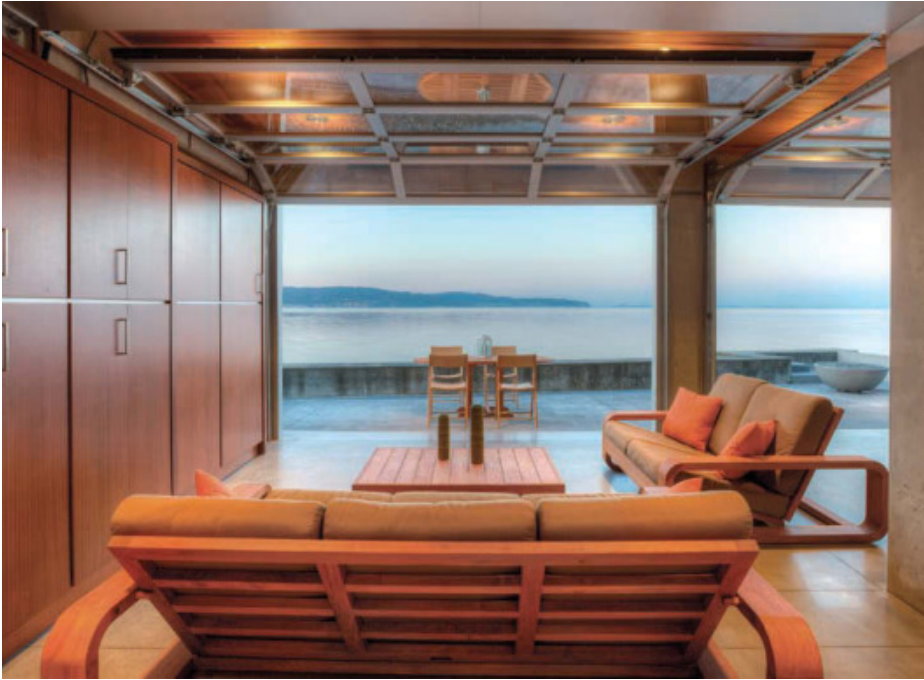
SIMPLICITY BELIES THE BUILD The open-air “Flood Room” on the lower level is both a tsunami solution and a peaceful respite. The walls and overhead garage doors are designed to break away if a tsunami hits, allowing water to flow through.
