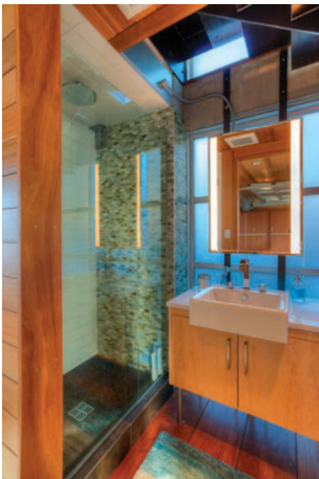
SMART STRUCTURE A translucent aluminum and frosted-glass wall allows for privacy and natural light.
