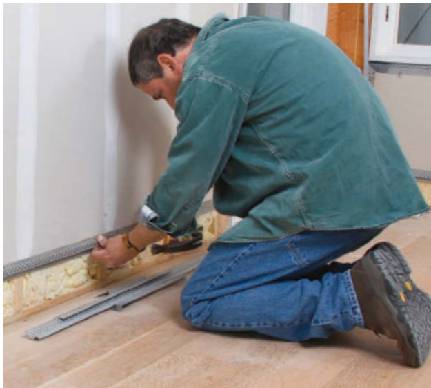
Case, then base. Once the window trim is complete, we install the trim for adjacent baseboard. When all the reglet is in place, we sand and finish the hardwood floors before the baseboard is installed.
