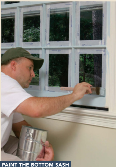
PAINT THE BOTTOM SASH
