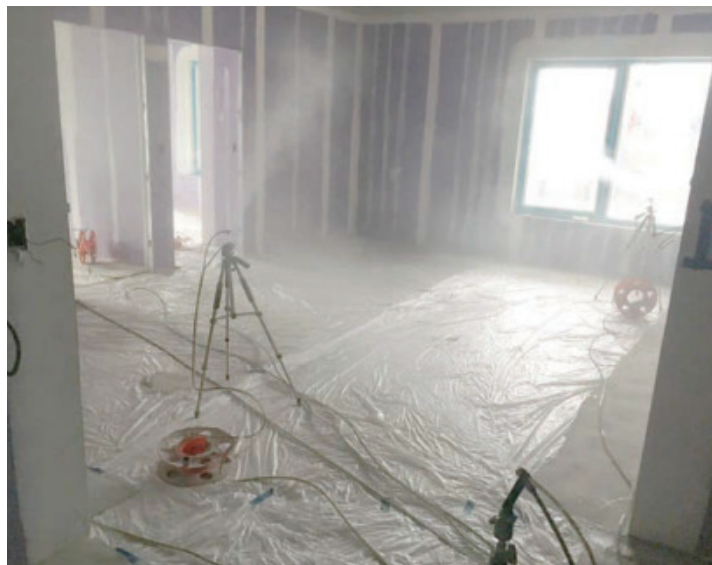
Spray air-sealing. AeroBarrier uses a series of emitters and pressure from a blower door to force a latex sealant into gaps and cracks in the building envelope. The process usually takes half a day or less.
