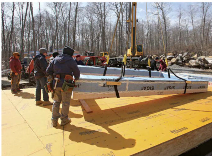
LANDING ZONE You'll need a flat location to set the panels after they are lifted off the truck. If you don't have a framed floor, make a suitable space on the ground.
