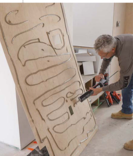
GLUE IT UP Use a construction adhesive like PL Premium to help hold the backing panels to the wall. This step helps eliminate any voids, hollows, or movement between the drywall and the plywood.
