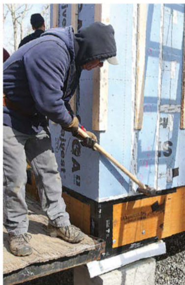
A LITTLE PERSUASION A skilled crane operator can get the panels very close to where they need to be. A sledgehammer helps nudge them the last little bit.
