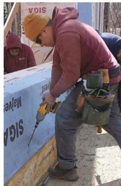
LOCATION, LOCATION, LOCATION Fastening locations are determined by the manufacturer, and the fasteners are all the same structural screws.
