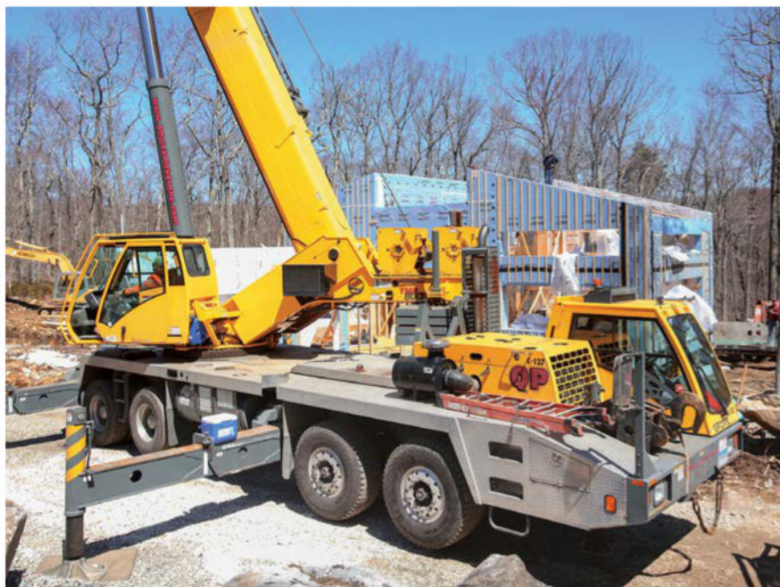
SIZE MATTERS The size of the crane is determined by the weight of the panels and the distance the crane needs to reach.
