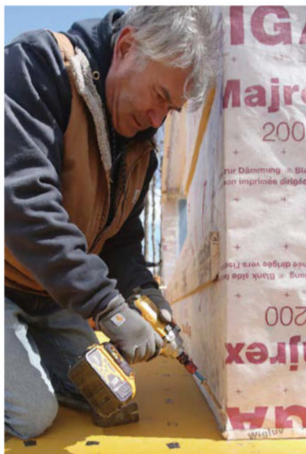
LOCATION, LOCATION, LOCATION Fastening locations are determined by the manufacturer, and the fasteners are all the same structural screws.
