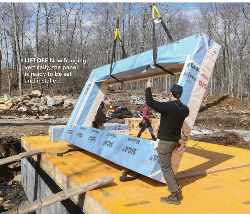
A BIT OF RE-RIGGING Brackets, blocking, and straps are removed, and the panels are re-rigged into setting position.
