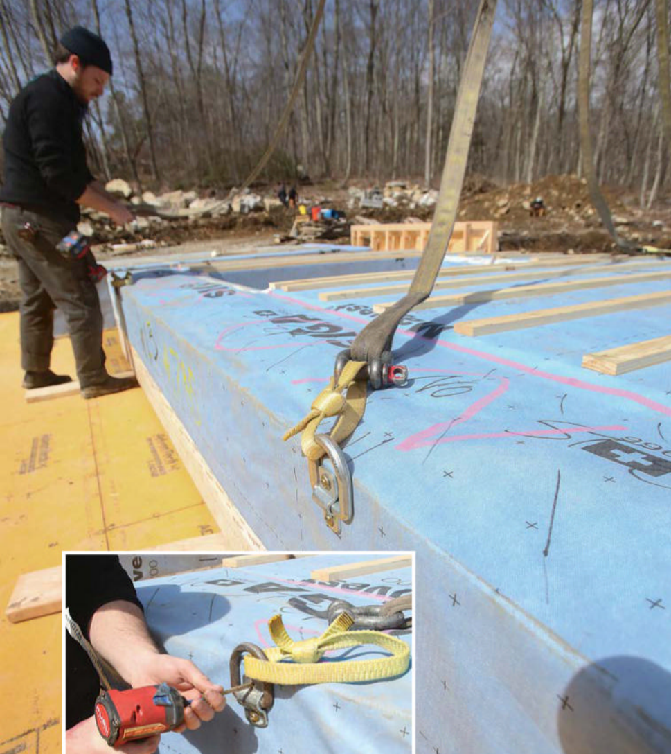
A BIT OF RE-RIGGING Brackets, blocking, and straps are removed, and the panels are re-rigged into setting position.
