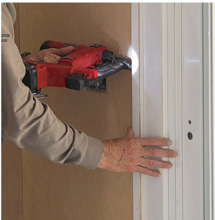
BRAD IN THE BACKBAND Cut any transition moldings to fit, such as the backband, and then send them home with an 18-ga. brad nailer.
