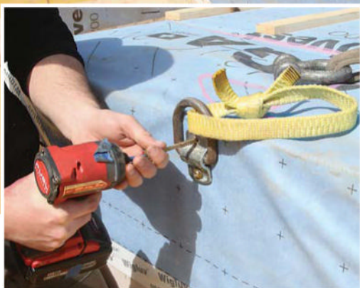
A BIT OF RE-RIGGING Brackets, blocking, and straps are removed, and the panels are re-rigged into setting position.
