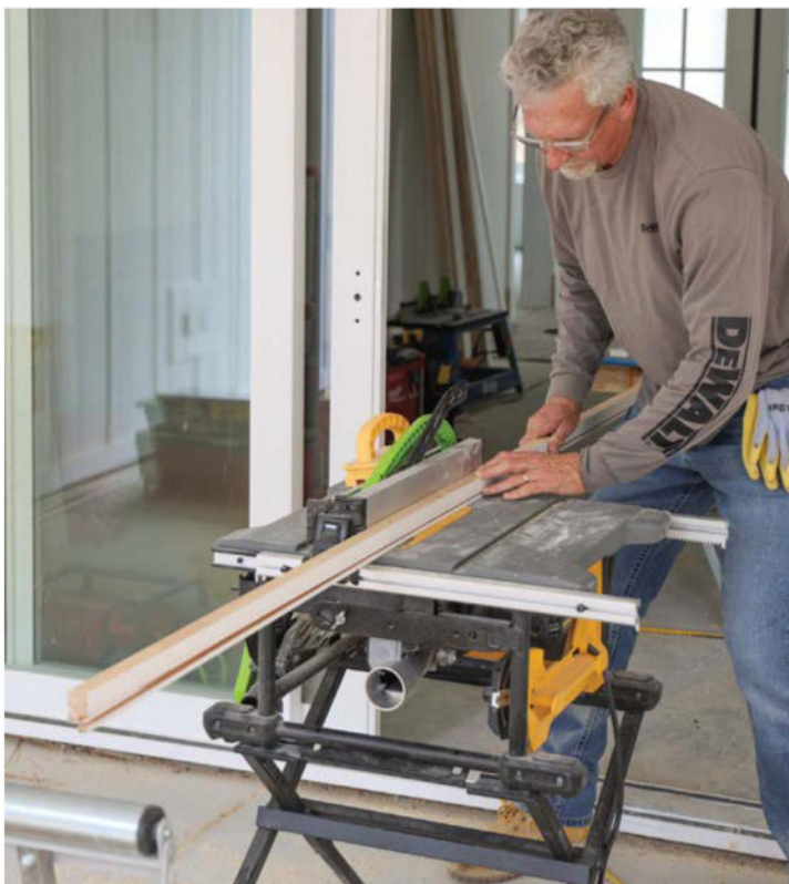
MILL THE CUSTOM MOLDINGS Using a tablesaw and a router, mill any custom-size moldings needed for the transition points, such as the backband.
