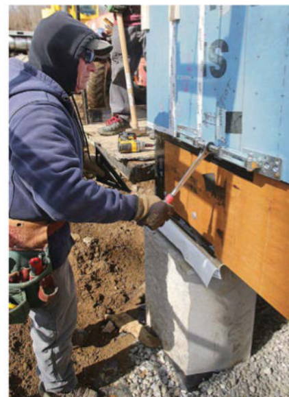
NICE AND TIGHT Ratcheting panel pullers are screwed to adjacent panels and used to pull them tight. When needed, the pullers can also be used to push panels where they need to go.
