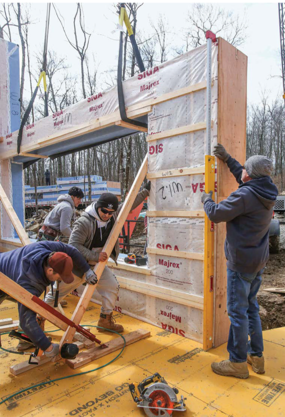
BRACING BASICS As with a stick-framed wall, the panels need to be braced plumb and straight before framing the second floor or stacking panels.
