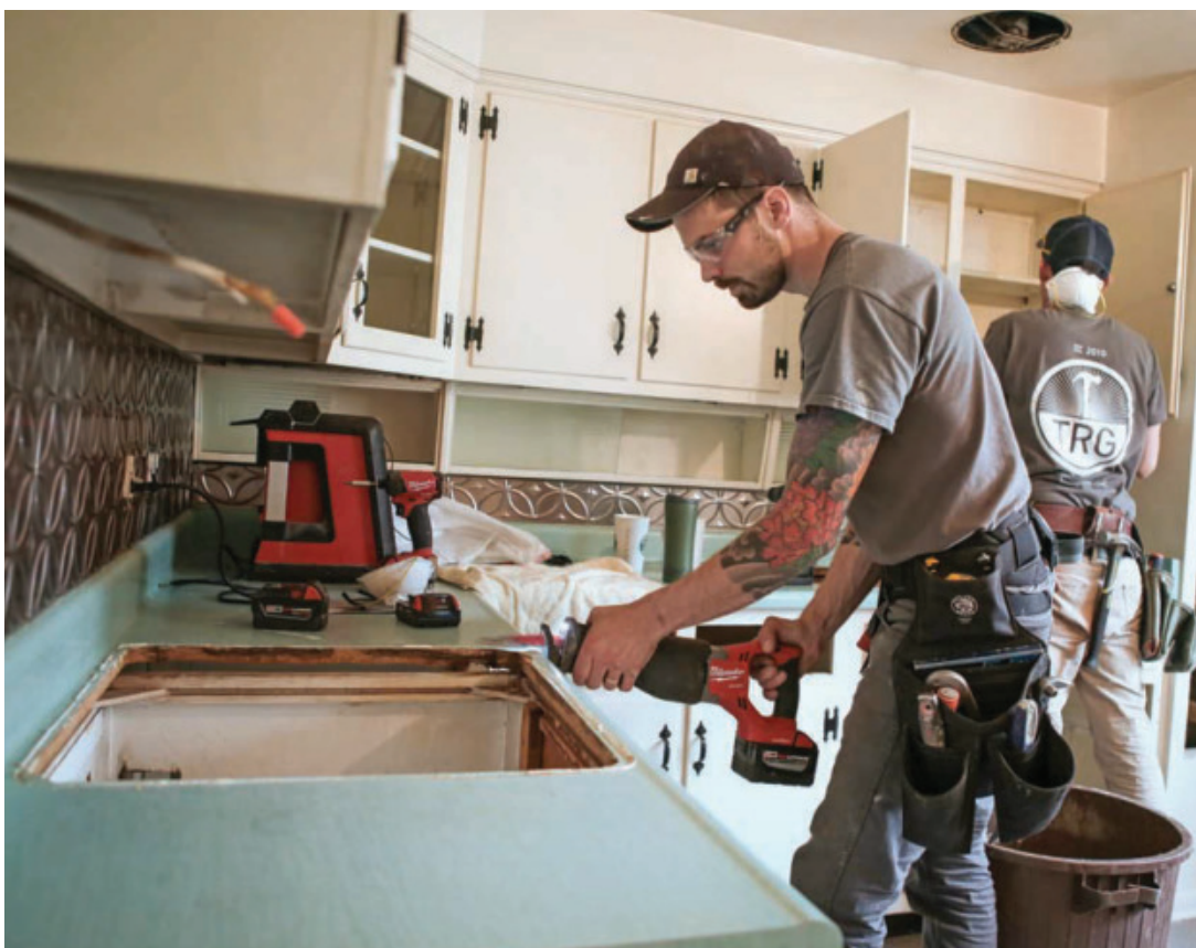
More real than reality TV. A snapshot from Tyler Grace's recent article demonstrates how a real carpenter handles demolition.
