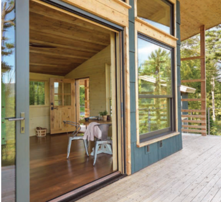
Natural cedar and painted pine. The decking and trim is all unfinished white cedar, which will age to a natural gray color. The unusually tall 20-in. painted shingles were hand-cut on site from white-pine slabs.
