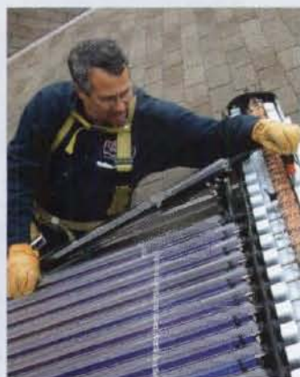
Liquid sunshine. The author assembles the Viessmann vacuum-tube solar array that produces 80% of the hot water for his home.
