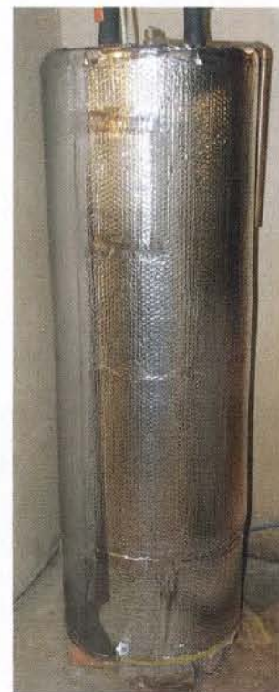
This insulation jacket from Energy Efficient Solutions ( www.energyefficientsolutions.com ) has an R-6 value and fits most tanks up to 80 gal.
