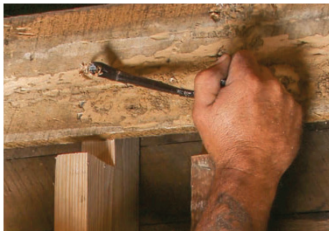
Cut the ribbon. Use a reciprocating saw to cut the old ribbon board on both ends and then use a cat's paw to remove the nails that hold it to the studs.
