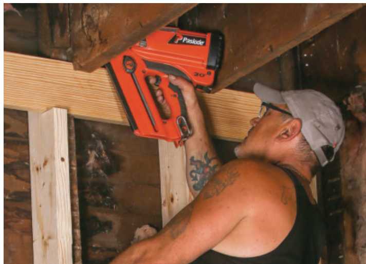
Attach the joists. When the floor is settled onto the new lower ribbon board, nail the joists to the sides of the studs.
