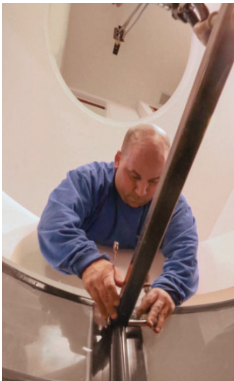
Preparing for lift. The hoist chain is attached to a temporary steel rod, which is fastened to a ring with metal pins.
