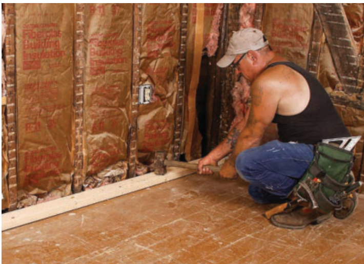
Gentle readjustment. A pair of heavyweight coworkers walking around or a board and sledgehammer lowers the ends of the floor joists, bringing them into contact with the ribbon board and making it level across the span.
