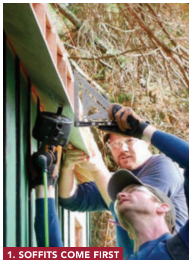
1. SOFFITS COME FIRST
