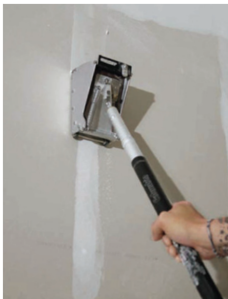
Spotters fill screws. Made in 2-in. and 3-in. widths, screw spotters are used to lay down a stripe of compound to cover drywall nails and screws.
