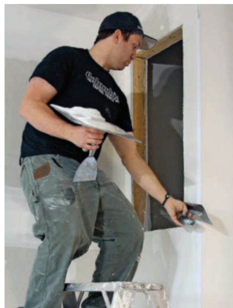
Handwork is still required. Automatic tools can finish a large part of the job, but you still need to know how to use hand tools for corner beads, repairs, and tight spots, like this AV equipment built-in.
