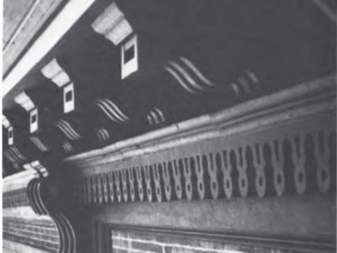
The Winooski Block (left) is capped by a cornice assembly over 6 ft. wide; it consists of 14 elements, including 7 moldings that were reproduced on a table saw. The milling of the molding is described on the facing page.
