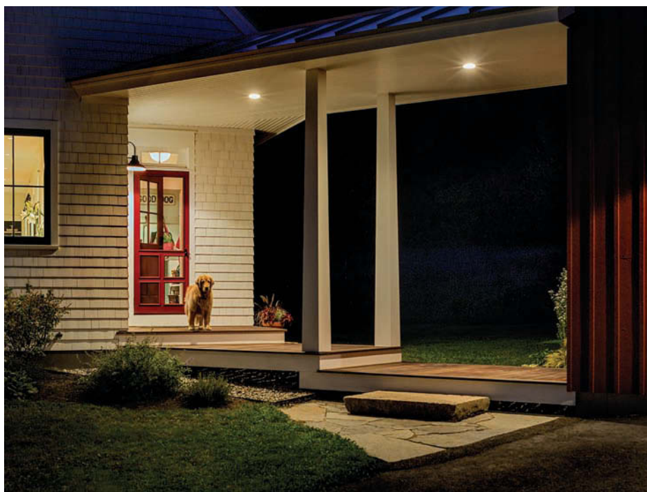
Covered connection. A sheltered walkway links the house's back entrance with the garage, about 20 ft. away. LVLs held up by tapered columns support the roof.
