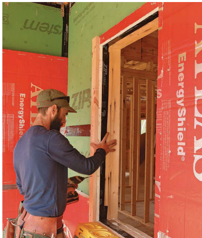
Install nailers. Screw rough-pine 5/4x3 nailers over the 1-in. foam to build the assembly out to the plane of the main 2-in. foam insulation.
