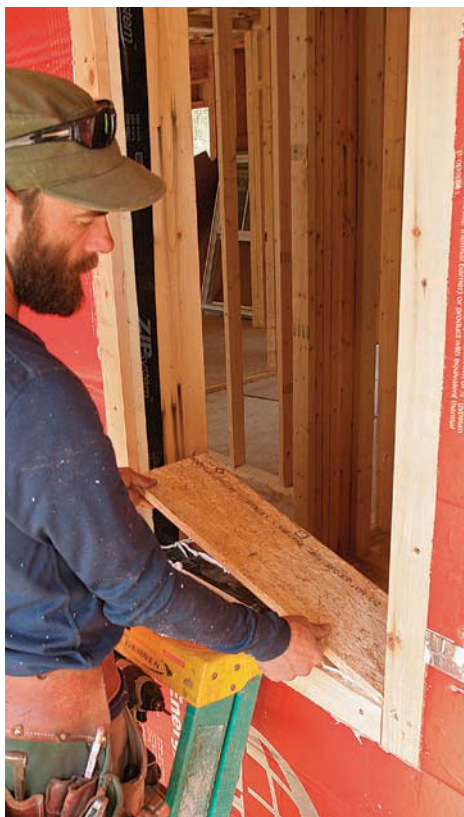
Add a solid sill. To create a base for windows and doors, fasten a piece of ¾-in. sheathing to the bottom of the rough openings.
