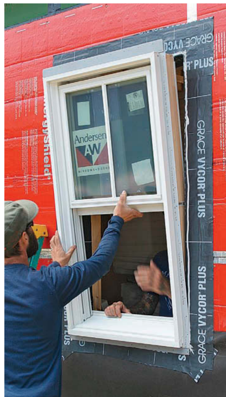
Proceed normally. With solid nailing established, installing windows or doors and integrating them with the WRB and the flashings is the same as on any other job.
