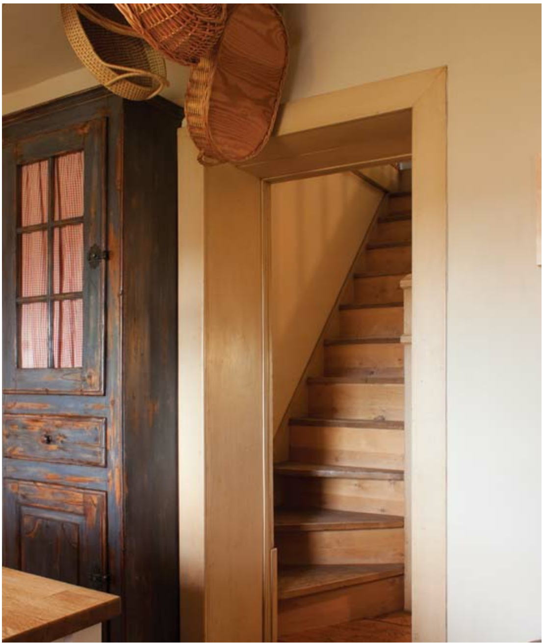
The staircase had been removed and covered up at one time; Lothar and Anita rebuilt it true to Early American—and European—forms.
