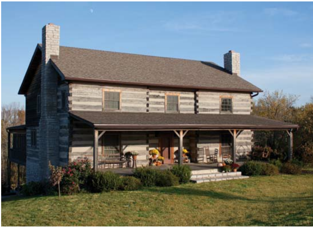
Middle Kentucky and Tennessee are well known for the unique style of hewn-log construction known as a “dog trot.”
