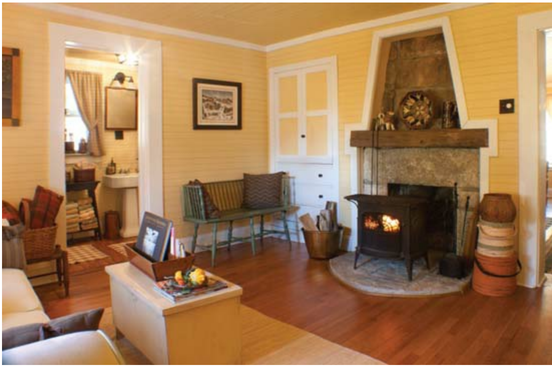
The early fireplace (made from quarried stone from the area) in this sitting room was an unexpected surprise—found in the restoration process.
