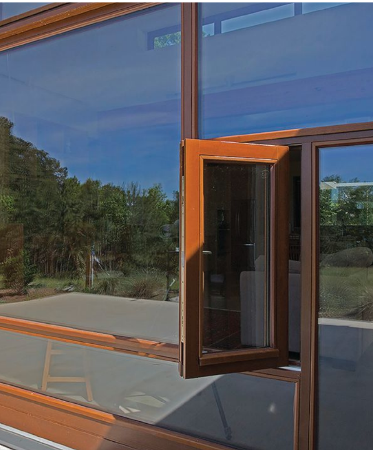
A wall of glass overlooking the courtyard shows off creative window composition. For maximum energy savings, Newphire Building sourced triple-pane windows from Europe.
