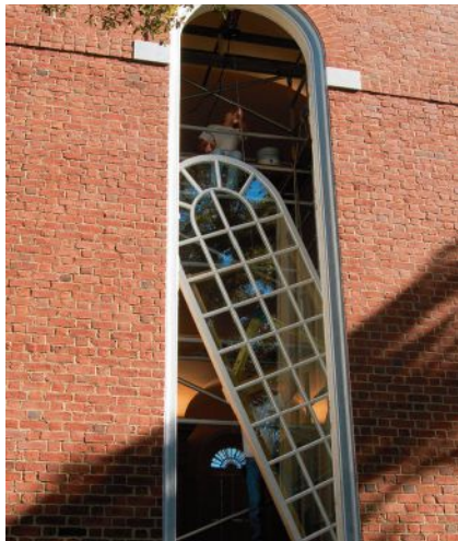
Counter clockwise from top: Completed windows weighed 700 pounds, challenging for transport and installation; the jig makes a concave cope cut on the end of the muntin bar where it meets the convex part of the inner arch; vertical muntins being notched, on a Laguna CNC; a concave cope cut lets the muntin meet the arch; gluing the lattice; profiling the convex side of the inner arch.
