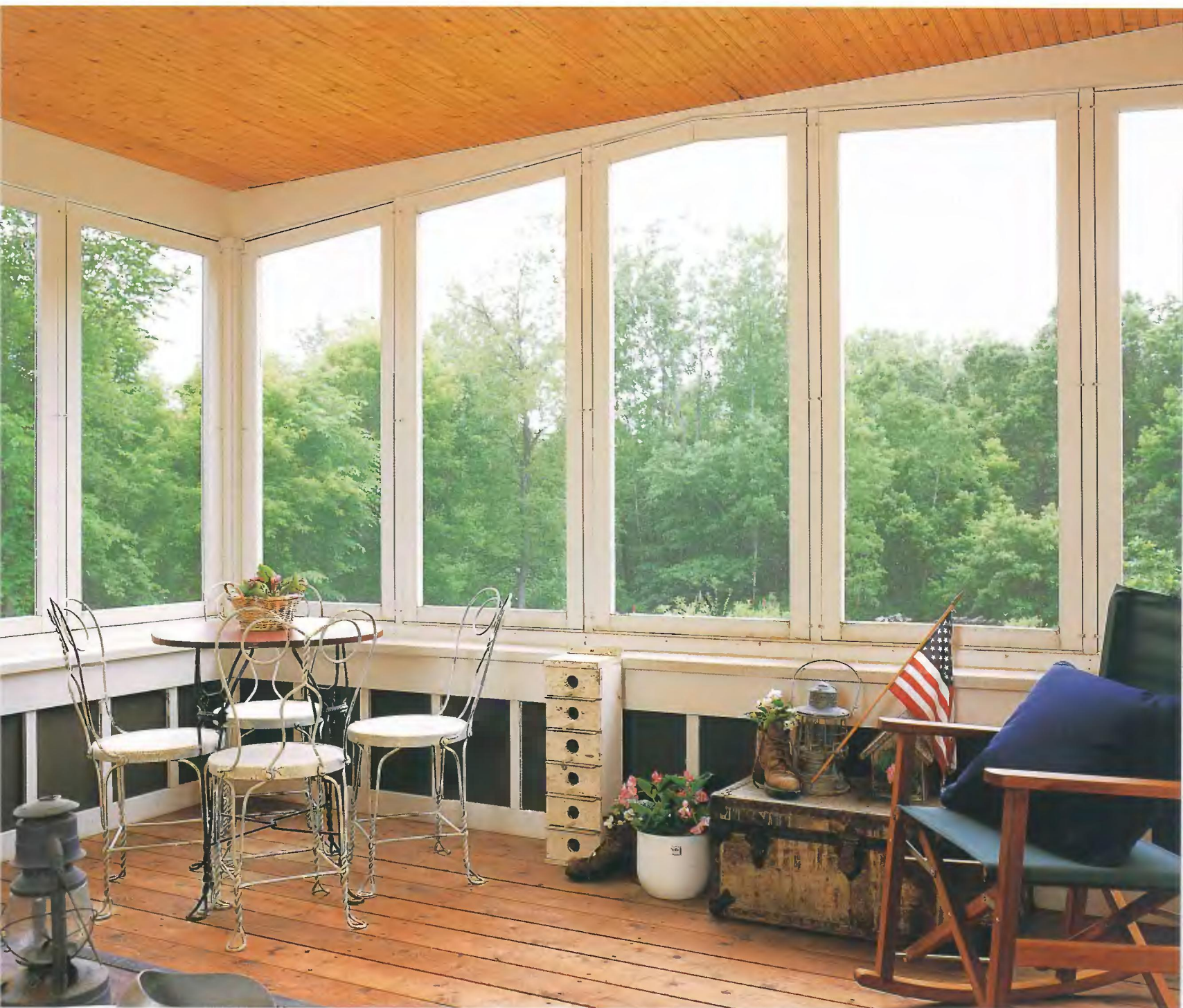
▲ The sleeping porch in this newly built Arts and Crafts-style home uses redwood flooring, which stands up well to humidity and moisture. The hardwood strips echo the linearity of the thin matchstick strips of the tongue-and-groove ceiling.
