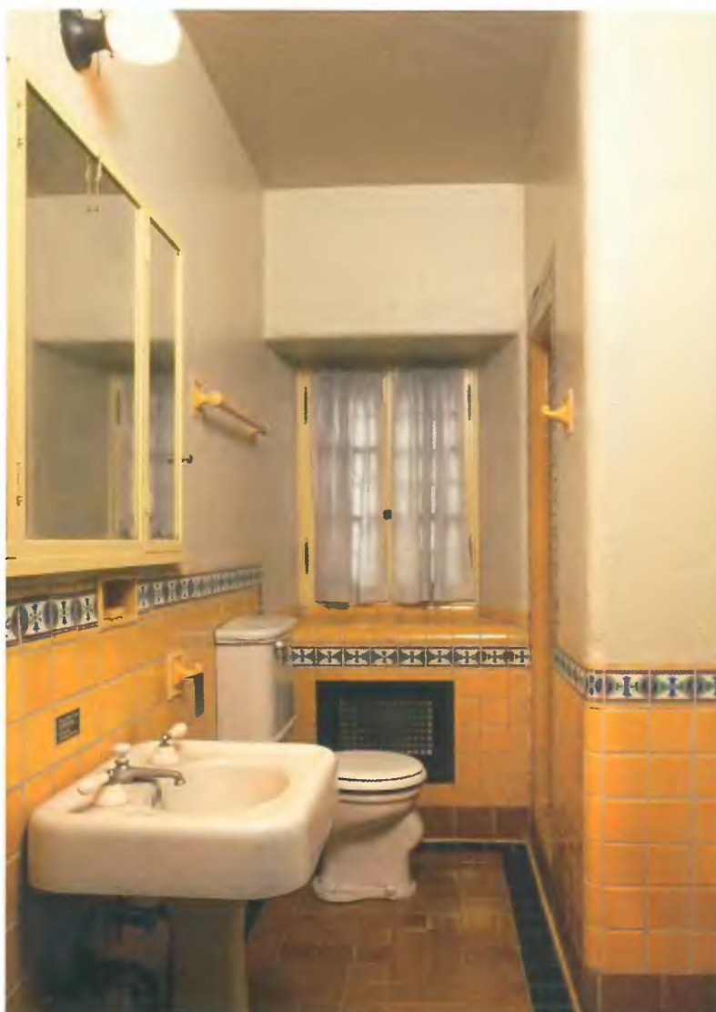
▲ This original bathroom with its striking tilework shows how little basic bathroom configurations have changed over the years. The layout features a pedestal sink with porcelain handles across from the bathtub. The bumped-out wall of the tub enclosure provides the space for a walk-in shower, just opposite the toilet.
