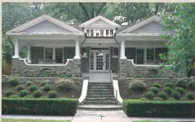
▲ The homeowners of this 1916 Washington, D.C., Bungalow replaced load-bearing walls with columns to open up the interior.
