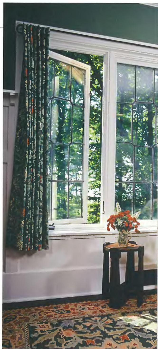
▲ Casement windows are often seen in Arts and Crafts and Bungalow homes. Here, glass panes are held in place with lead muntins, complementing the geometry of the wall paneling. Photo © www.carolynbates.com , Sandra Vitzthum Architect, LLC.
