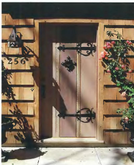
▲ A board-and-batten door with elaborate wrought-iron strap hinges reflects the intricacies of ironwork characteristic of Mission-inspired Bungalows. Photo © www.carolynbates.com , Sandra Vitzthum Architect, LLC.
