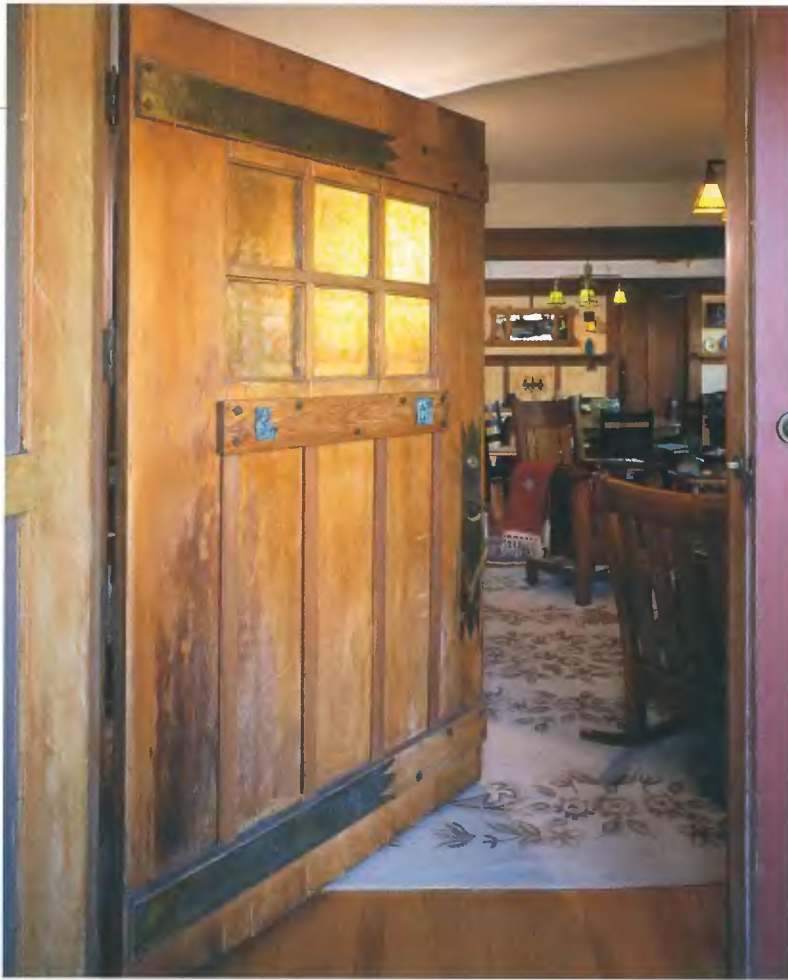
▲ Taking cues from a cabinet door on the original built-in sideboard in the dining room, a replacement door features overscaled strap hinges and a colorful art-glass upper panel.
