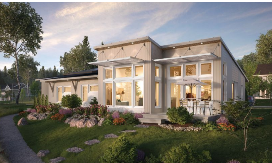
Unity Homes woodworker Tristan Pozo readies timber beams for assembly at Unity Homes' Walpole, N.H., factory. Below, a rendering of the Greenbuild Unity Home exterior.
