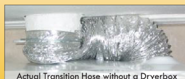
Actual Transition Hose without a Dryerbox
