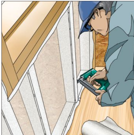
1. Net the Framing Cavities
