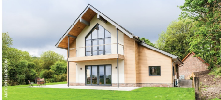
Above: Steve and Dory Morris took a truly hands-on route to their self build, even designing the house themselves using SketchUp ( www.sketchup.com ). They opted for a structural insulated panel system for the main shell, partly because their contact at SIPs Eco Panels ( www.sipecopanels.co.uk ) provided helpful design suggestions. The couple took up references for suppliers and trades, which paid dividends throughout the project. The only real issues came with the plasterers and renderers, who were messy and difficult to manage. "The other tradesmen were good as gold," says Steve. The 375m 2 house was completed for £376,000.
