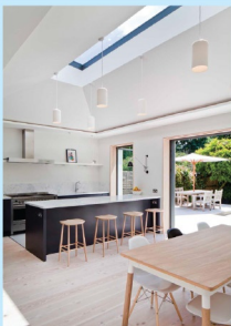
This extension includes a 3,780mm-long bespoke skylight that helps to throw light deeper into the kitchen. The Aero Electric unit by Sunsquare is operated by remote and has a rain sensor for peace of mind
