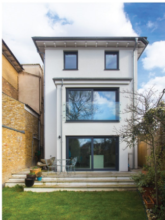
Above and above right: This stunning home is actually a new end-of-terrace infill on a brownfield plot in south west London. Owner Matt Warnes used a prefabricated timber frame building system from Hanse Haus ( www.hanse-haus.co.uk ) for a quick construction schedule that would minimise disruption to neighbours. The house is clad in characterful brick slips that help it blend into its surroundings
