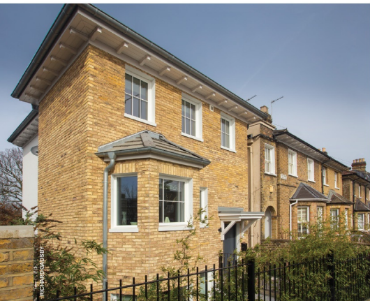
Above and above right: This stunning home is actually a new end-of-terrace infill on a brownfield plot in south west London. Owner Matt Warnes used a prefabricated timber frame building system from Hanse Haus ( www.hanse-haus.co.uk ) for a quick construction schedule that would minimise disruption to neighbours. The house is clad in characterful brick slips that help it blend into its surroundings
