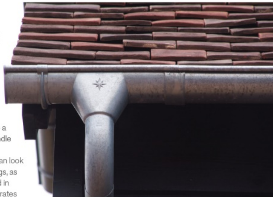
Above: Stainless steel guttering, such as this version from Yeoman Rainguard, is highly resistant to corrosion, making it a robust choice for homes subject to the worst of the British weather
