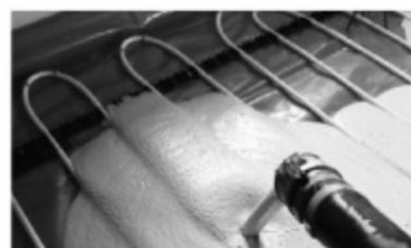
Liquid screed being poured over UFH pipe installation
