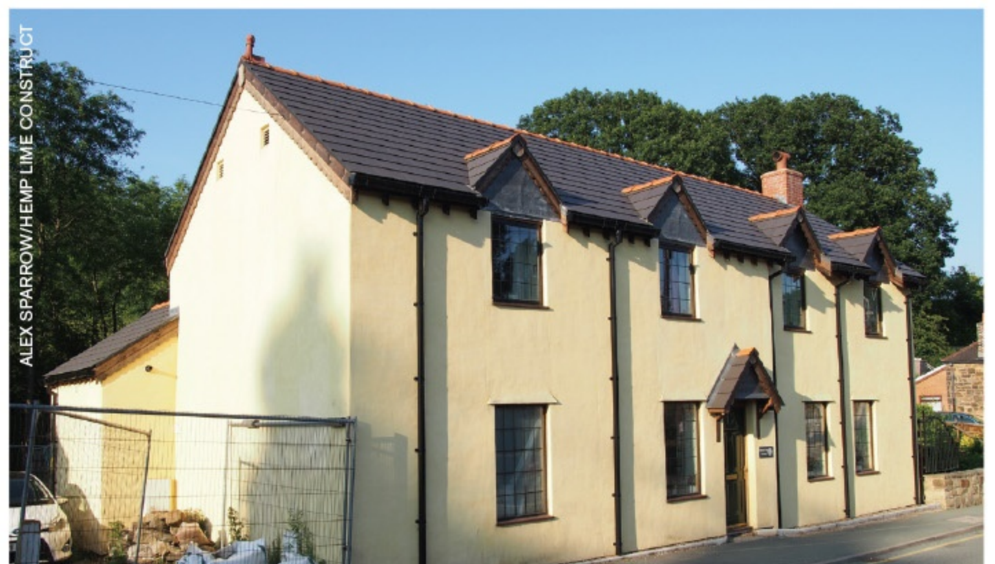
Victorian cottages restored by a self builder, who cast hempcrete external solid wall insulation from Hemp Lime Construct as a new cladding
