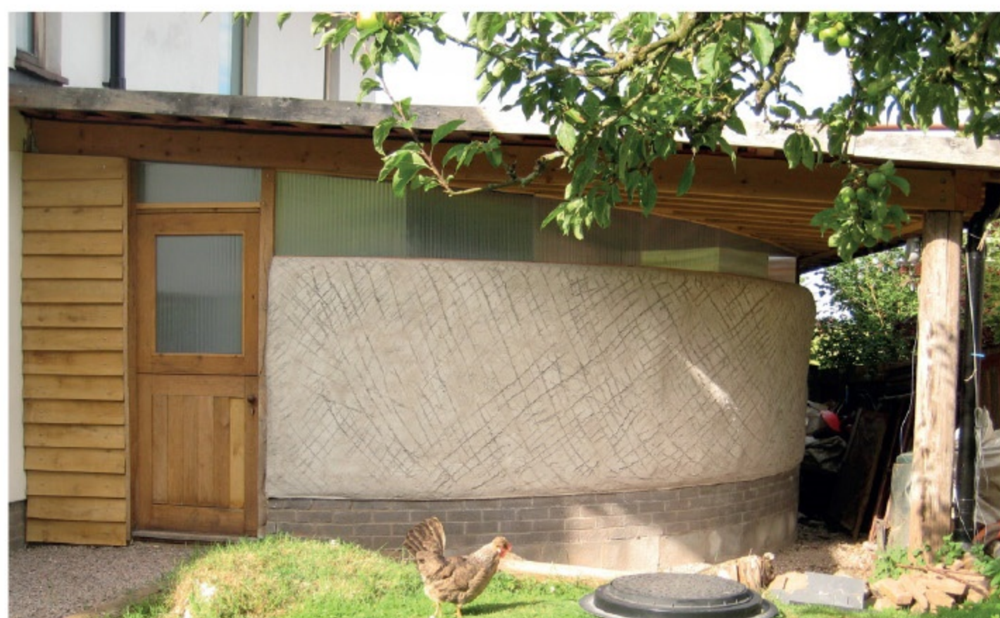
Top left: Husband-and-wife architects Steven Harris and Catherine Roberts of CRSH Architects tried out straw bale construction by building their garage-workshop with a curved wall under a large projecting roof. Top right: The garage has the first of its lime render coats and will eventually be painted. Above: The finished structure
