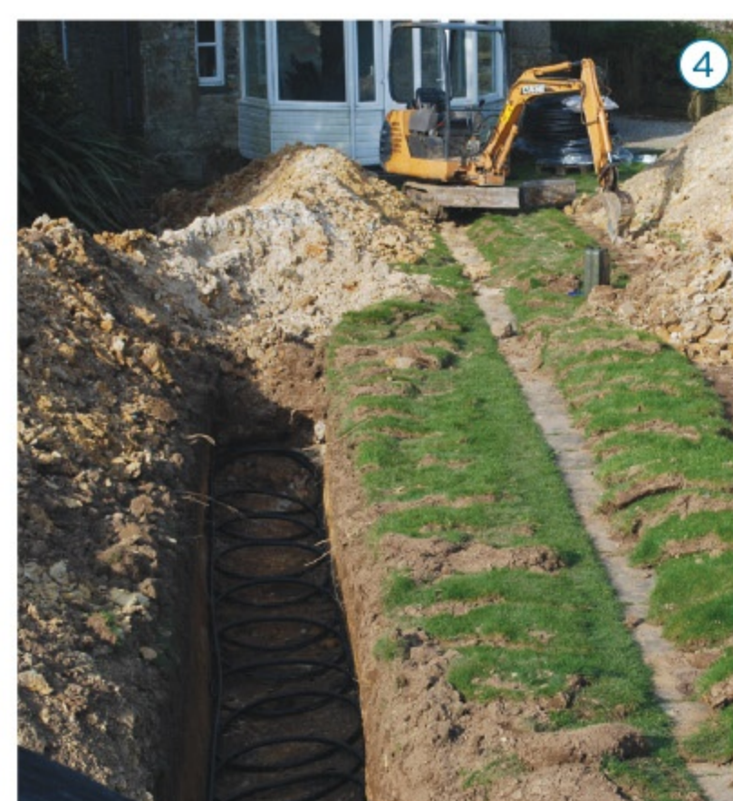
1 Manifolds for the underfloor heating are concealed in the lower part of an old door opening in the living room 2 The tank for the heat pump is fitted 3 To compensate for the vaulted ceiling Stephen installed Celotex insulation above Building Regs standards 4 The coils for the pump get laid in the garden
