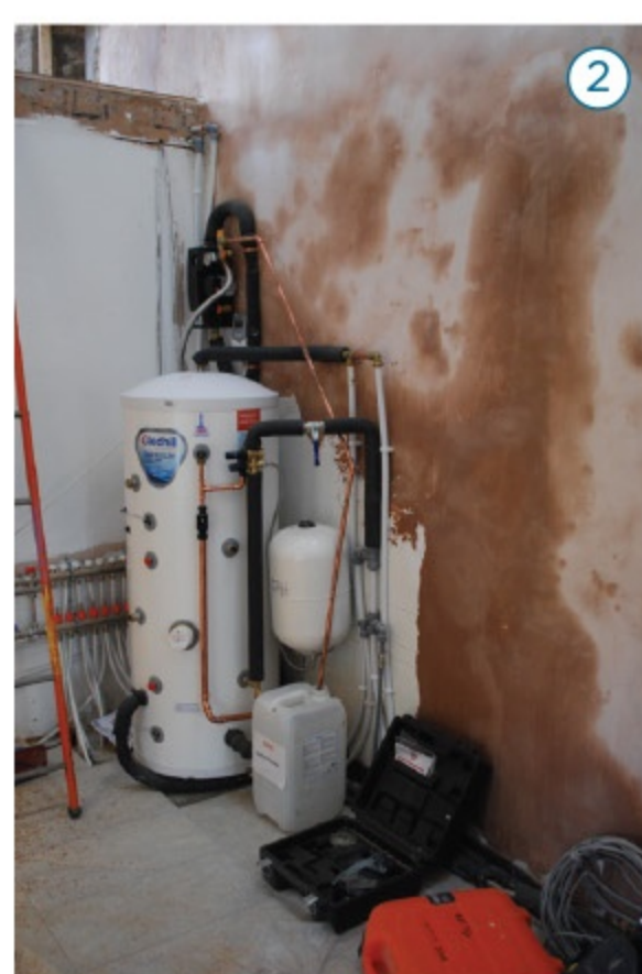
1 Manifolds for the underfloor heating are concealed in the lower part of an old door opening in the living room 2 The tank for the heat pump is fitted 3 To compensate for the vaulted ceiling Stephen installed Celotex insulation above Building Regs standards 4 The coils for the pump get laid in the garden
