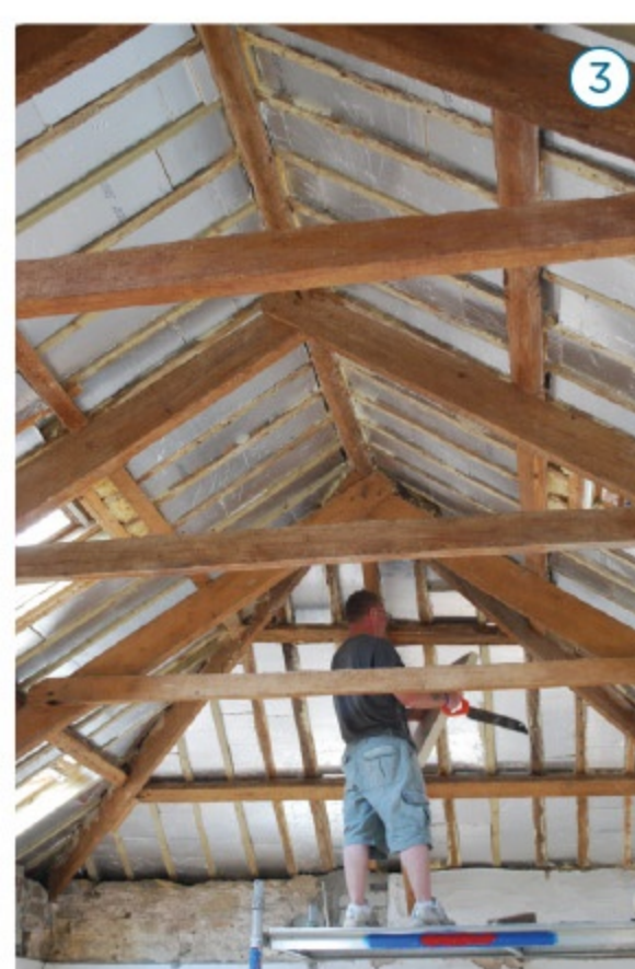
1 Manifolds for the underfloor heating are concealed in the lower part of an old door opening in the living room 2 The tank for the heat pump is fitted 3 To compensate for the vaulted ceiling Stephen installed Celotex insulation above Building Regs standards 4 The coils for the pump get laid in the garden
