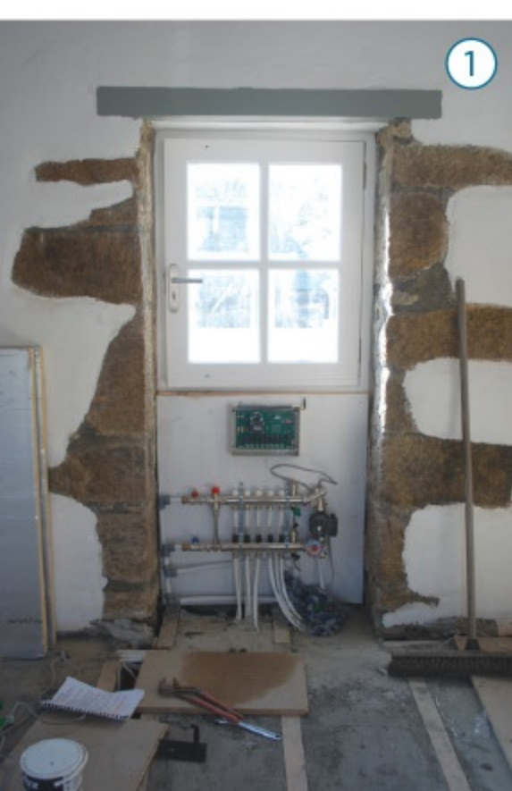
1 Manifolds for the underfloor heating are concealed in the lower part of an old door opening in the living room 2 The tank for the heat pump is fitted 3 To compensate for the vaulted ceiling Stephen installed Celotex insulation above Building Regs standards 4 The coils for the pump get laid in the garden
