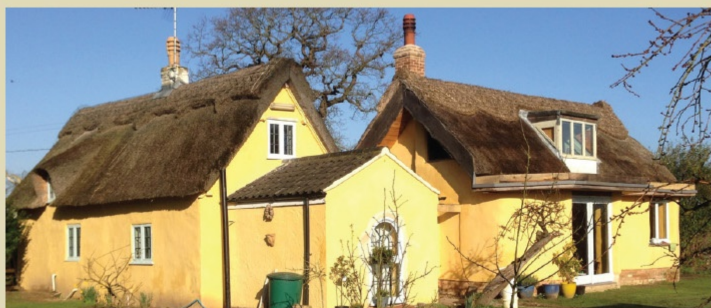
An original 'clay lump' house, extended with cob and straw bale, with a cob staircase and fireplace inside. The project, carried out by Edwards & Eve Cob Building, doubled the size of the cottage for just £10,000
