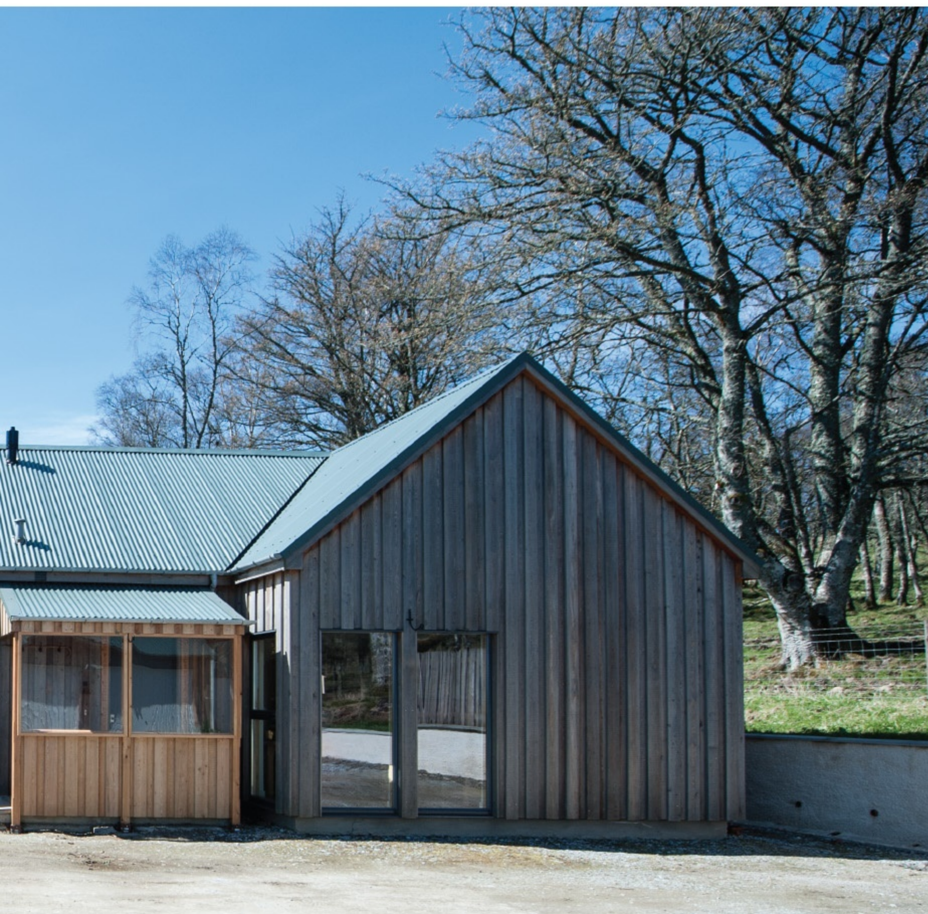
Left: From the side, the full view of the new extension, which is completely hidden from the road, is revealed. The porch leading to the boot room is a newer addition, built by Alastair himself
