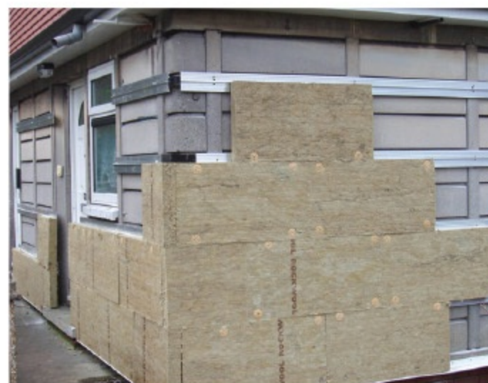
Insulating solid walls externally (in this case with rockwool batts) is a great way to improve a home's overall thermal performance at the same time as updating its appearance
