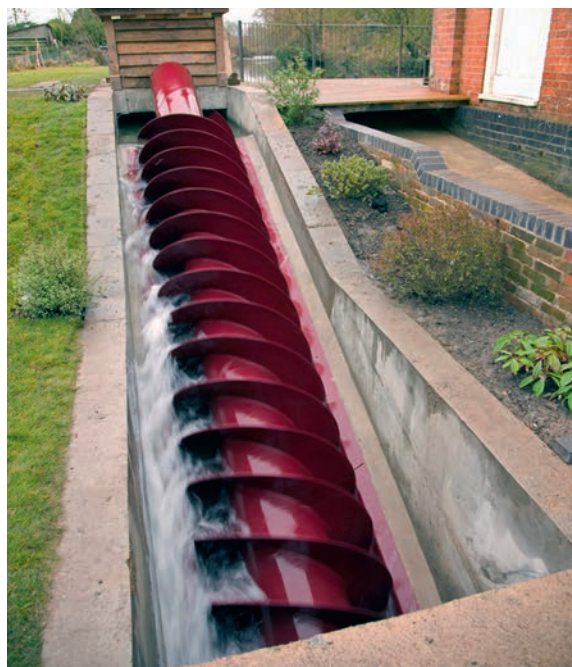
Left: LAPD Architects utilised an Archimedes screw as part of their strategy to generate energy from the waterway on this site
