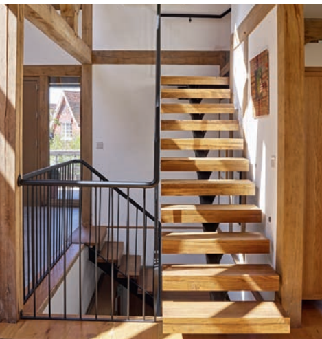
Above: This home by Welsh Oak Frame is perfectly complemented by the modern timber and cast iron staircase. The open treads are supported by a robust central spine that matches the balustrade
