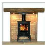
Chop into an existing chimney breast
