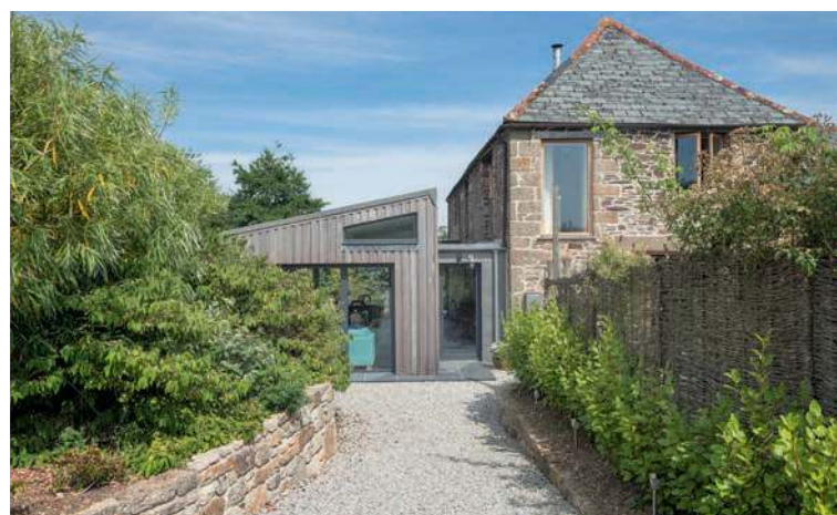
Above: The cedar cladding on the extension helps form a clear visual distinction between the new addition and the original stone barn
