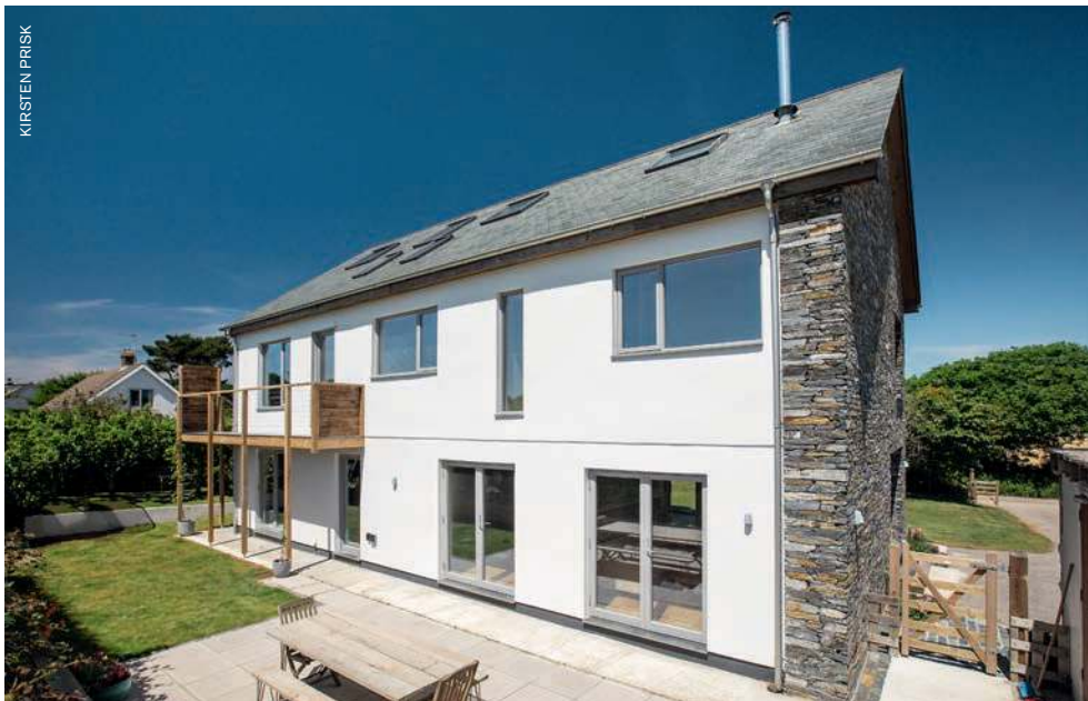
Above: Even though neighbours objected to the proposed height of this project, built on a street full of bungalows, Barry and Jenny Tape managed to get planning permission within five short weeks
