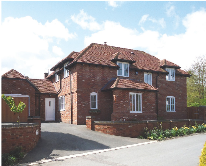
Left: This 180m 2 family home by Design & Materials blends in with the village scene. Built in masonry with solid floors and walls throughout, it achieves a U-value of 0.17 W/m 2 K for the external walls
