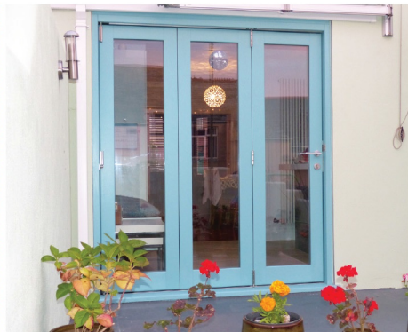
Above: These Kloeber timber doors in cheerful sky blue were specified for a seaside location. The company recommends that any timber products in a coastal setting are recoated more frequently than ones in a less harsh environment, and it also offers a marine-grade finish on aluminium products for an additional cost
