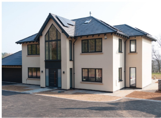
Above: This contemporary turnkey self build project by CB Homes features an internal leaf of insulating blockwork, followed by 100mm of cavity wall insulation, an external skin of solid concrete block and a render finish. The 262m 2 house (plus 37m 2 garage) achieved a high B-rating on its energy performance certificate (EPC), and is fitted with a heat pump, solar panels, underfloor heating and triple glazing
