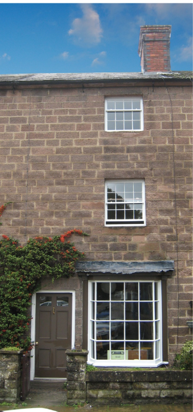
Above and right: This cottage is part of a world heritage site, set within a conservation area and listed to boot – but Alan Tierney and his team still managed to achieve a high-quality renovation that balances modern life with the building's original character; and reinstate some lost features along the way
