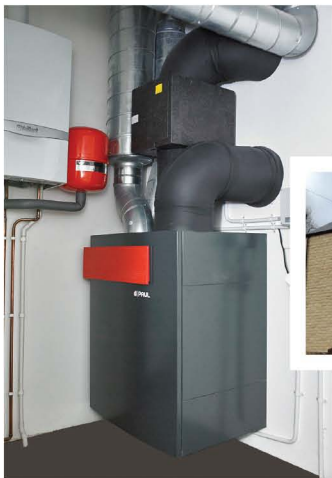
Left and above: This Passivhaus in Golcar, Yorkshire, features a Novus 300 MVHR unit by Paul, supplied by the Green Building Store, housed in an upstairs plant room. The system cost £5,000 and works in tandem with a gas boiler to provide efficient warmth for the 261m 2 property
