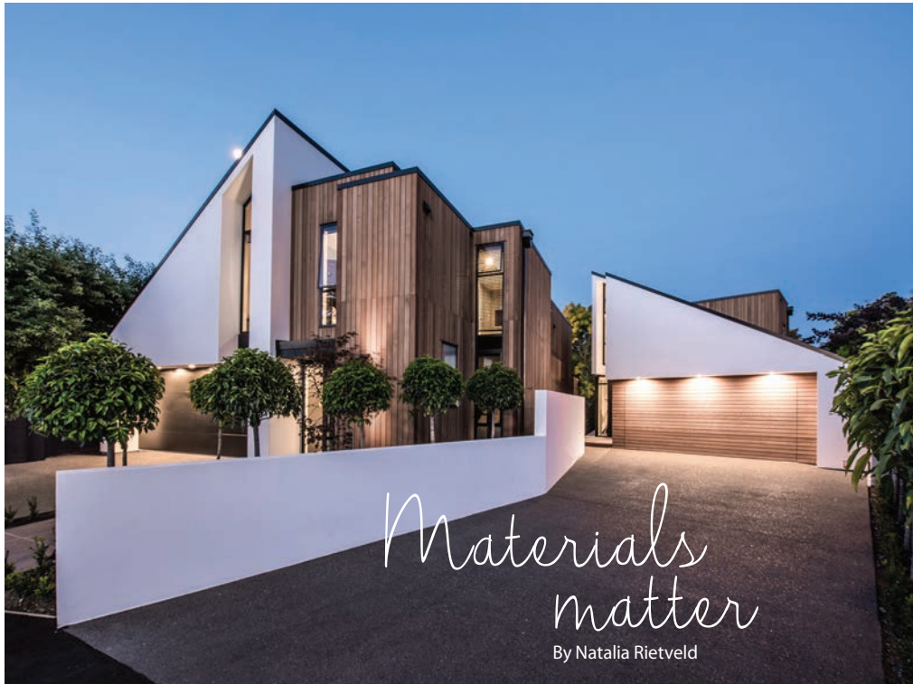
Gleneagles Terrace, designed by Craig South of Cymon Allfrey Architects.
