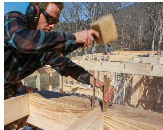
Shims for the tenons. Untapered oak shims draw the shoulders of the joists tight against the beam face, locking the joists into place.
