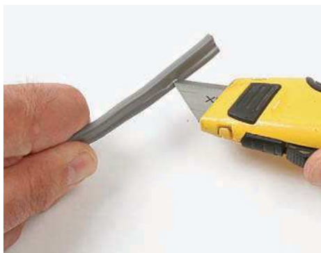
Cut down the UF-B cable's concave center.
