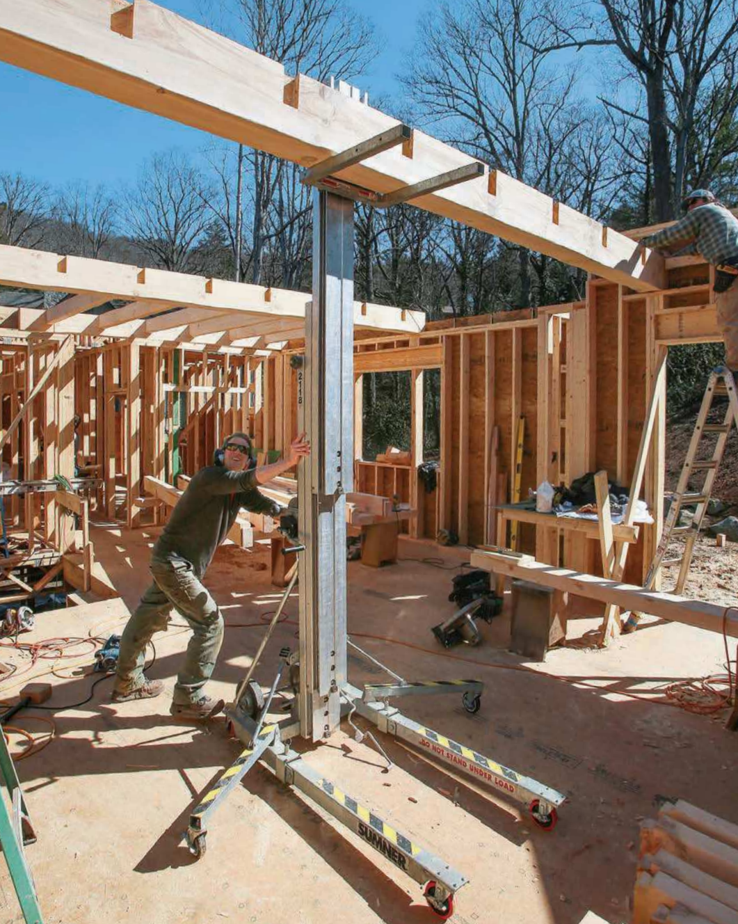
Easy lifting. A wheeled material lift, available from rental yards for about $60 a day, makes quick work of lifting the beams and joists into position.
