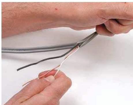
Pull the conductors out from the jacket.
