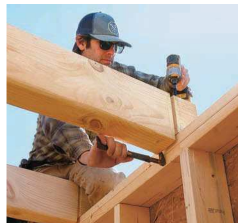
Screws for the plates. With the drywall groove aligned to the interior face of the stud wall, a single structural screw (TimberLoks were used here) driven through the top of its end secures the joist to the top plate below. Because the lumber is wet, no pilot hole is needed.
