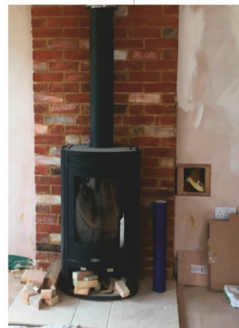
FINAL INSPECTION Ian employed a HETAS-certified professional to install his woodburning stove — ensuring it received sign off during the final inspection from the building control officer.
