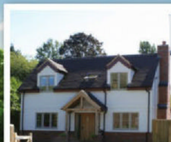
NEW BUILD HOME
