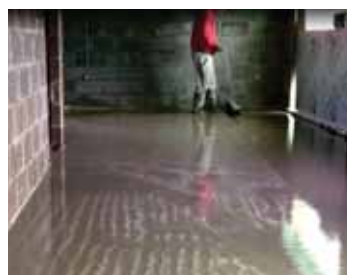
10 The final process is tamping the screed.
