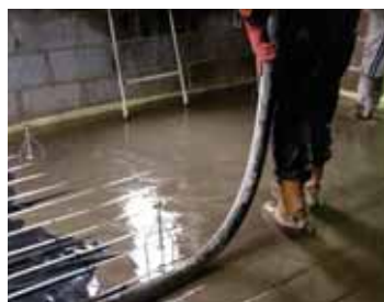
8 Self-levelling screed is carefully poured over secured pipe work.
