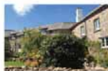
Renovation - Air Source
