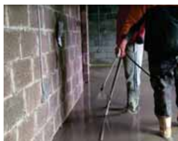
9 Screed is stabilised with chemical spray.
