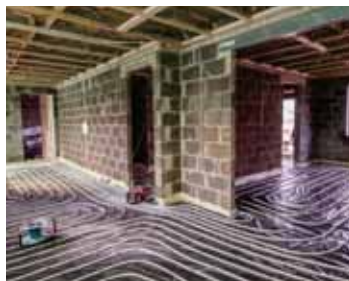
5 The pipe is all laid out. Multiple loops can make up a large space.
