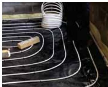
4 The pipe is then fixed at correct spacing.
