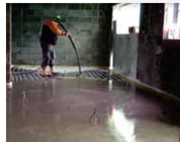
7 Screed is poured to the correct depth.
