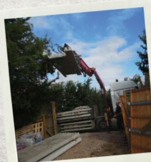
Each 'bundle' of beams weighed 750kg.
