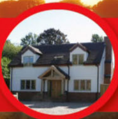
New Build Home
