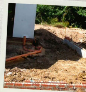
Builder Godfrey had to modify the drain run.
