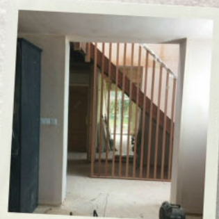
Sapele spindles run to the floor on the new staircase.
