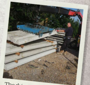
The driver was able to stack the beams out of the way.
