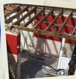
The rear of the house was completely stripped back.
