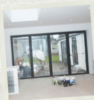
Bifold doors and a rooflight bring light into the extension.
