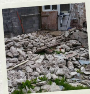
Part of the existing extension was demolished.
