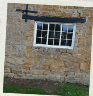
Dressed stone was needed to repair the external walls.
