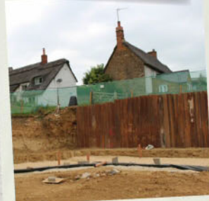
Charlie could have saved money on his sheet piling.
