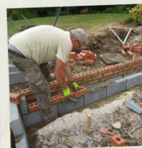
The brickies began work on the lower walls.
