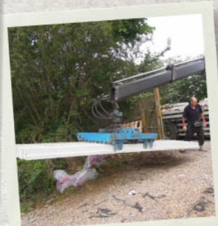
52 beams had to be craned onto the site.
