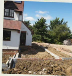
The site, ready for the delivery of the beams.
