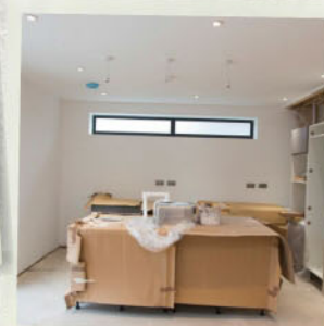
Fitting the kitchen is the next job.
