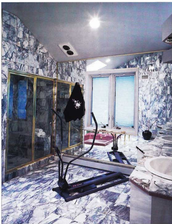
▲ Since it is prone to stains, marble tile must be sealed when used in the bathroom or other wet areas.
