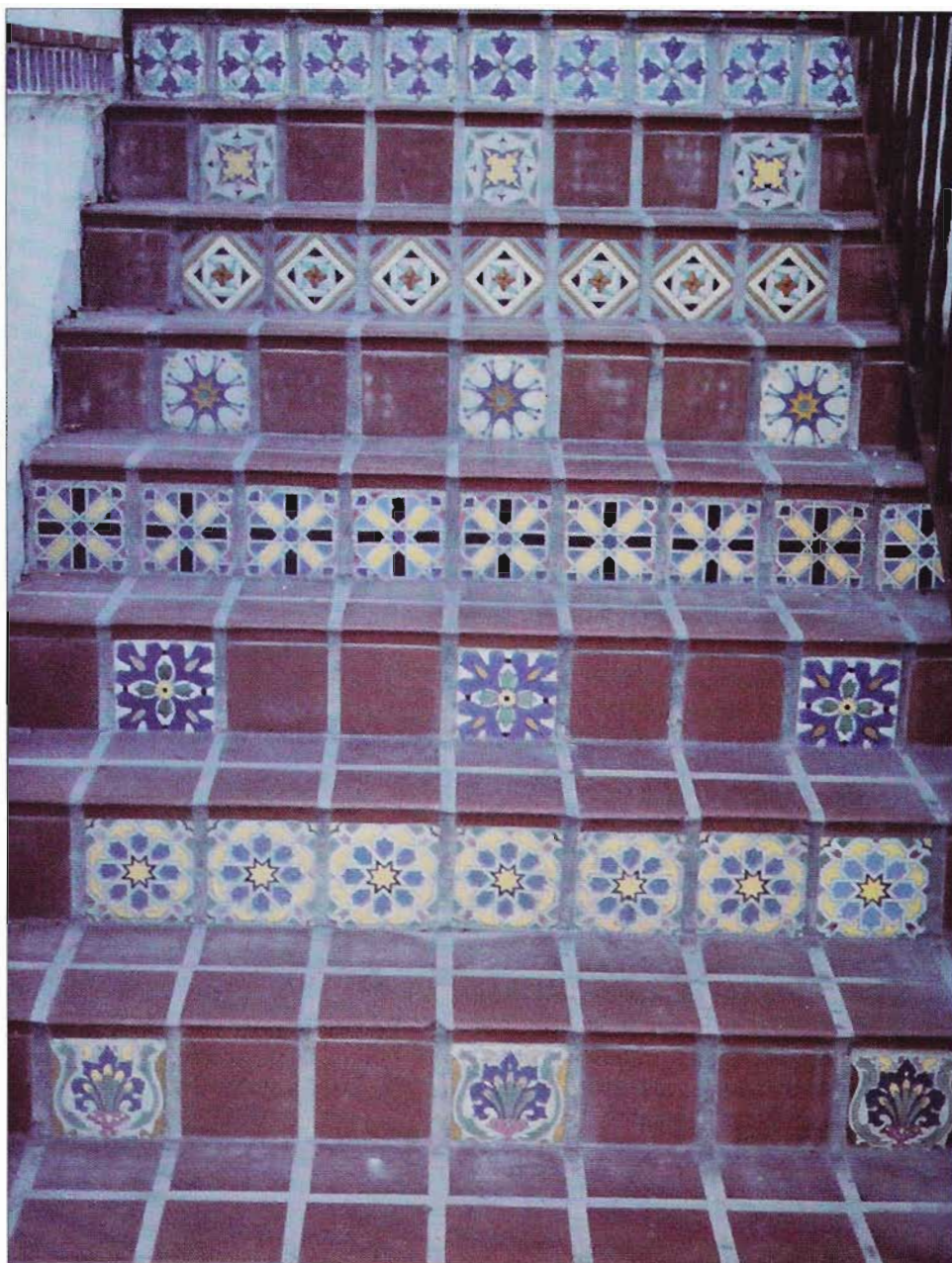
▲ Be sure to choose non-skid tiles when tiling stair treads.
