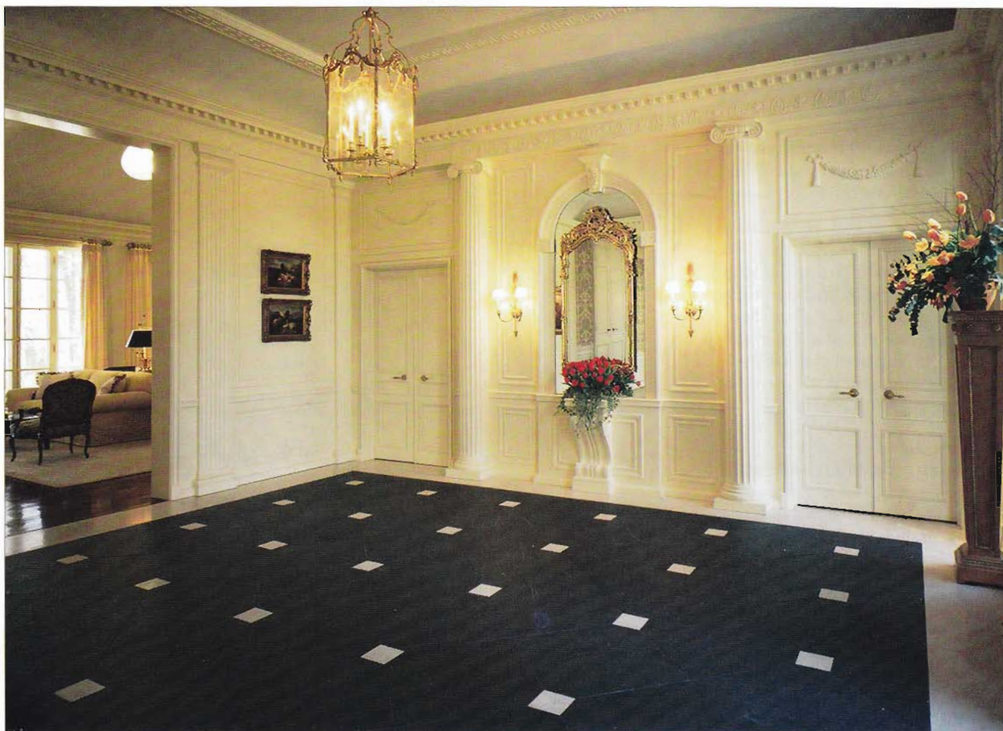
▲ Machine-gauged slate tiles are uniform in thickness and can be installed like other stone tiles.
