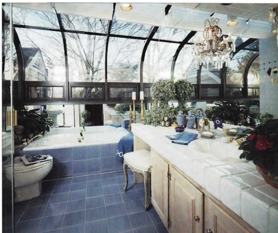
▲ The same tile that is used on the floor can be run up the side of the tub. Garden windows allow an exceptional amount of light to enter.
