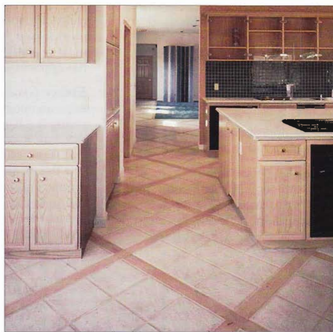
▲ Use your imagination when creating a floor pattern. Here, wood planks were used as borders for slightly undulated tiles.
