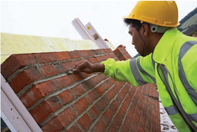
▲ Figure 4.36 Take the time to produce a joint finish to a high standard
