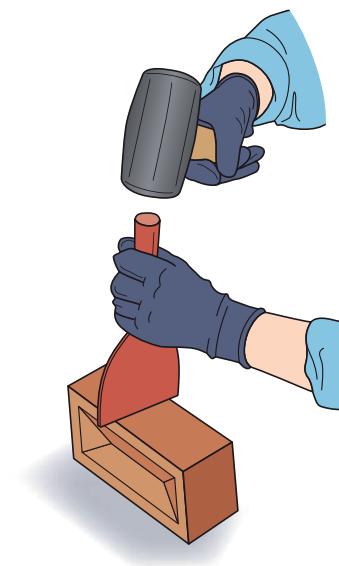
▲ Figure 5.28 A club hammer and brick bolster are used to cut bricks
