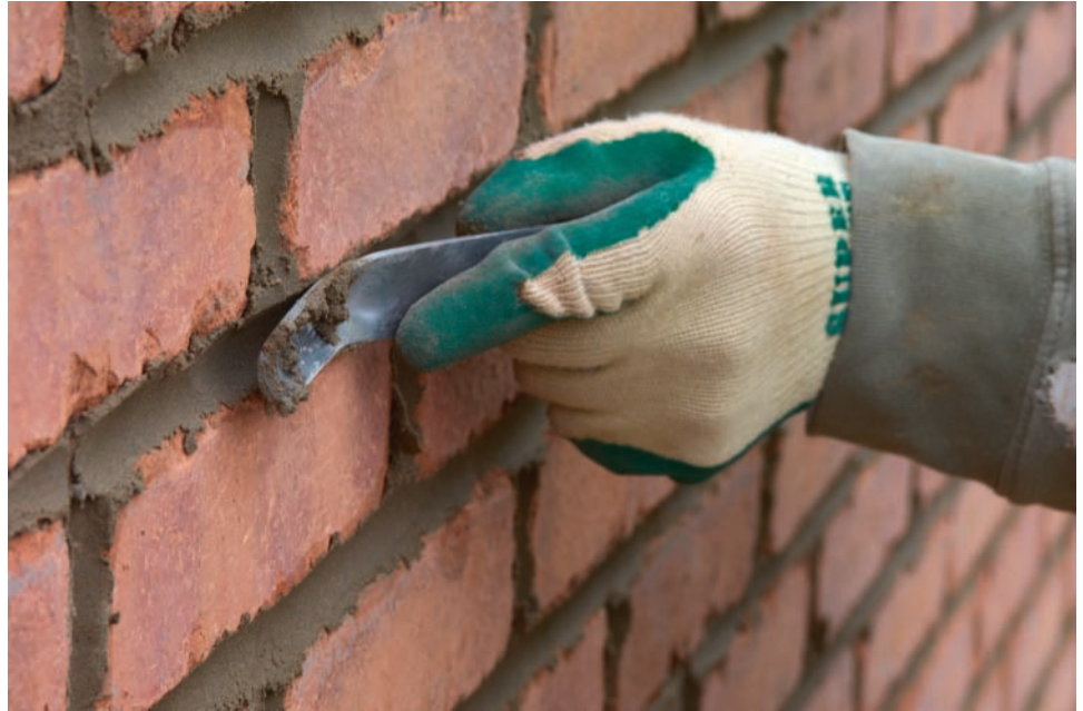
▲ Figure 5.43 Ironing the mortar joints to seal them
