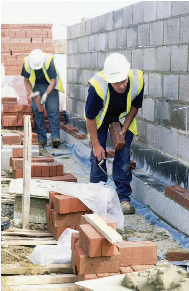
▲ Figure 5.37 Bricklayers laying to the line
