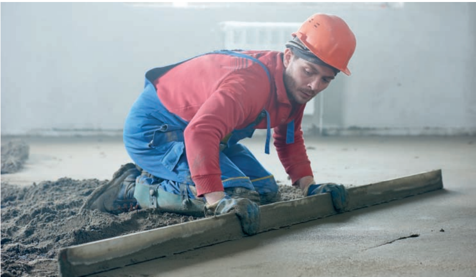
▲ Figure 1.27 Laying a screed finish to a solid concrete floor
