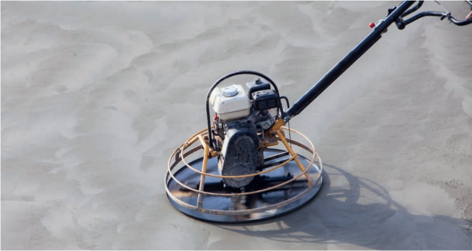
▲ Figure 1.26 Providing a smooth finish to a solid concrete floor
