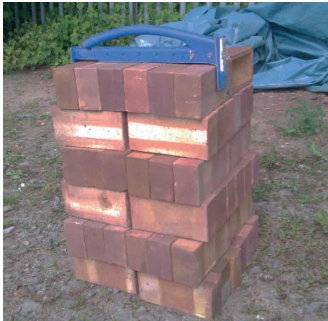
▲ Figure 5.20 Bricks stacked properly (note the use of the proper tool for moving bricks)
