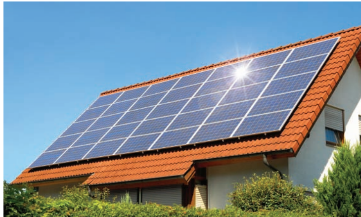
▲ Figure 1.14 Solar panels
