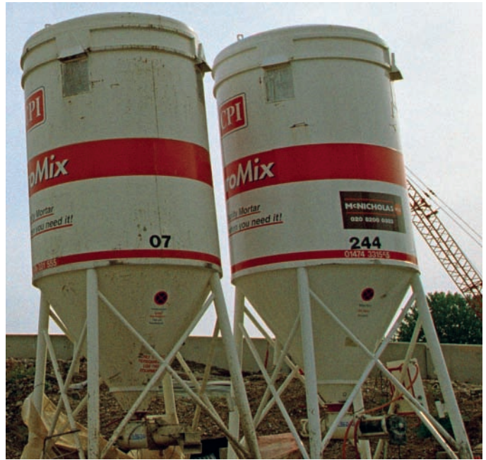
▲ Figure 3.19 Dry silo mixers
