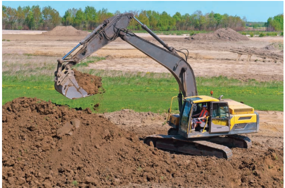
▲ Figure 2.3 Removing topsoil
