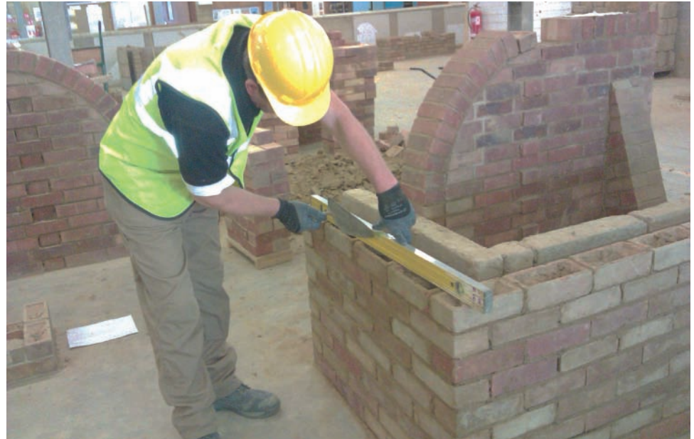
▲ Figure 5.30 Spirit level being used to level the top course of brickwork
