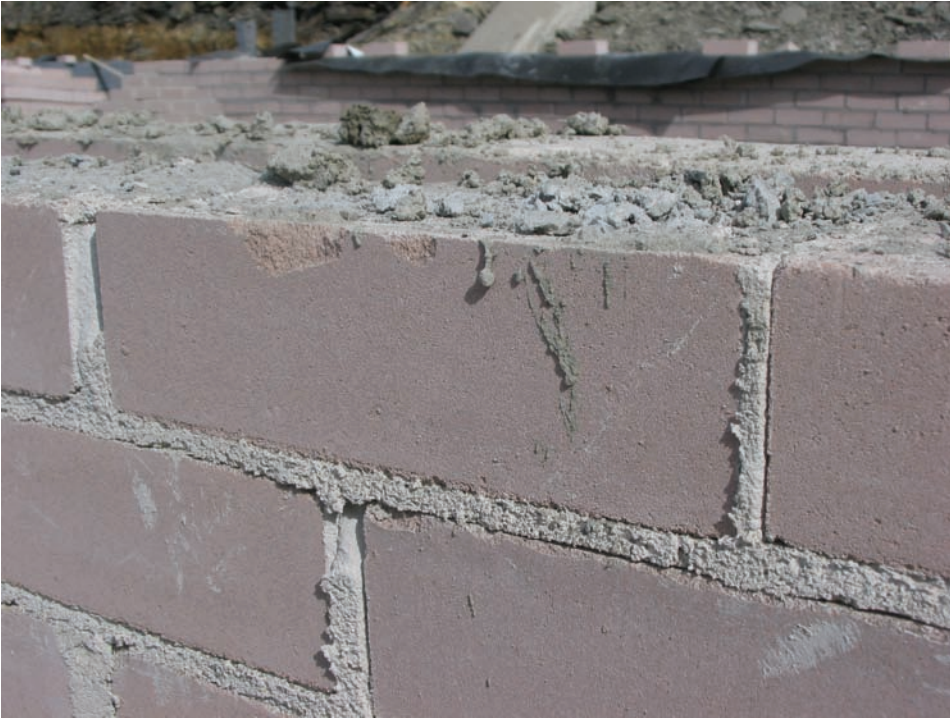
▲ Figure 5.11 A sand/lime brick wall
