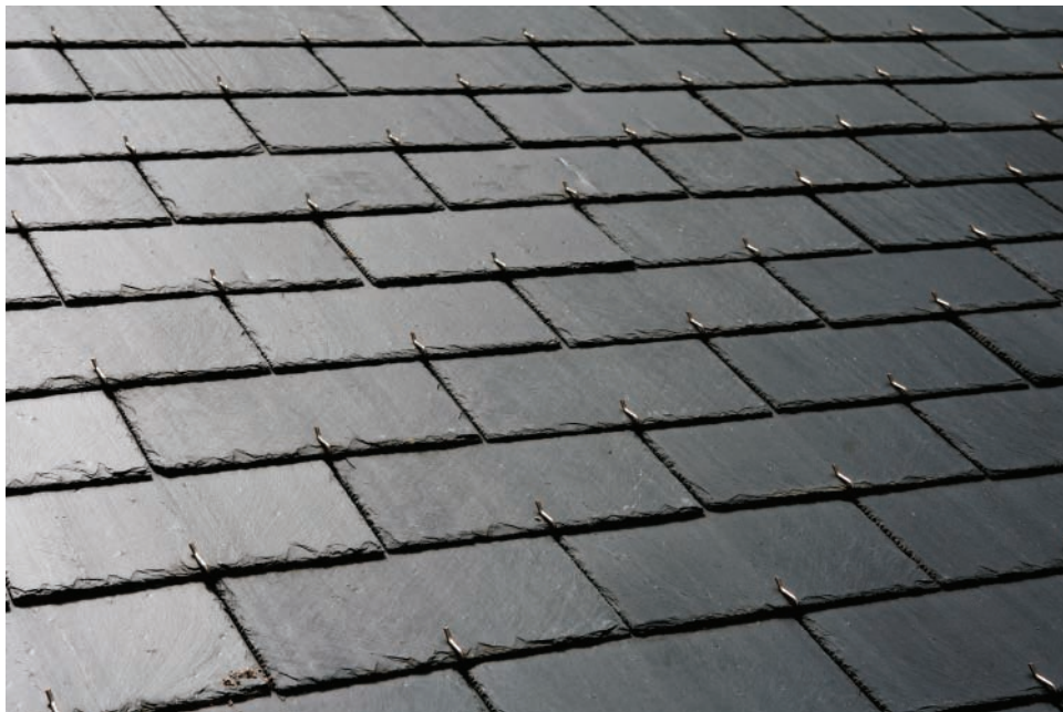
▲ Figure 1.46 Natural slate roof covering
