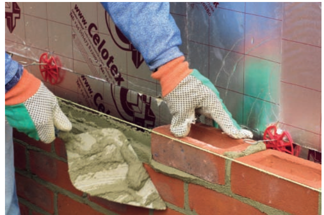
▲ Figure 4.31 Laying to the line
