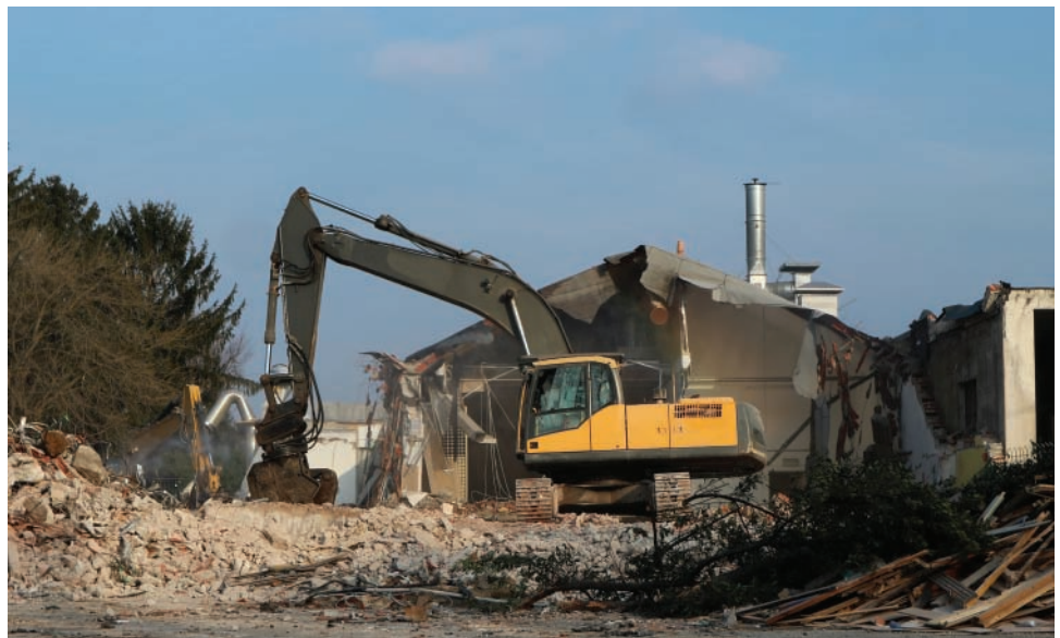
▲ Figure 2.4 Clearing a site of existing buildings
