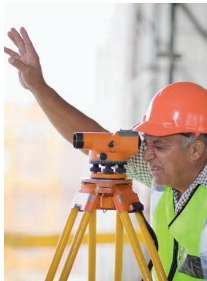
▲ Figure 2.25 One operative takes a height reading with the optical level
