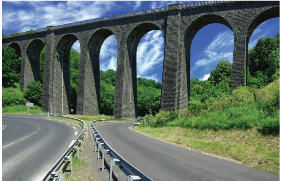
▲ Figure 5.13 A railway bridge built with engineering bricks
