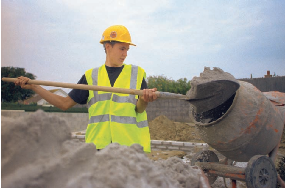
▲ Figure 4.15 Getting the right mortar consistency takes practice
