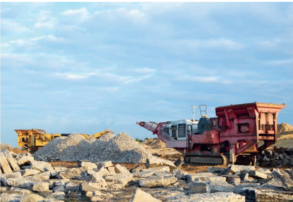
▲ Figure 1.21 Concrete can be crushed and recycled
