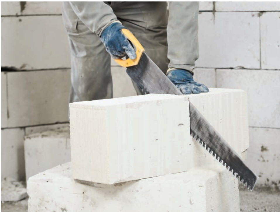
▲ Figure 3.31 Cutting lightweight insulation blocks with a hand masonry saw
