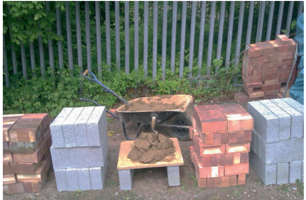
▲ Figure 5.22 Bricks, blocks and mortar ready for use to build a cavity wall on site
