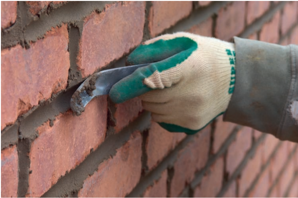
▲ Figure 4.35 Ironing the mortar joints to seal them
