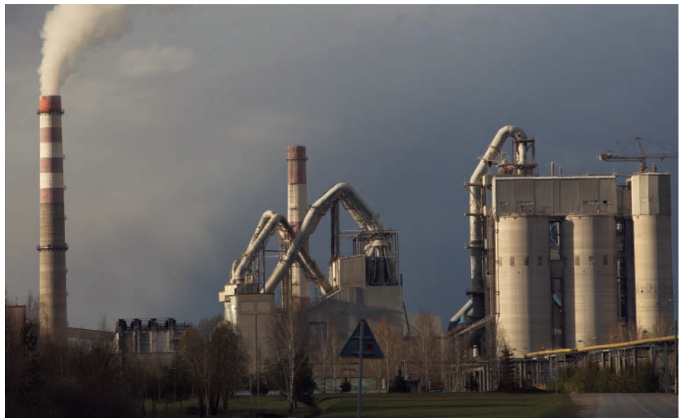
▲ Figure 1.19 Concrete production plant
