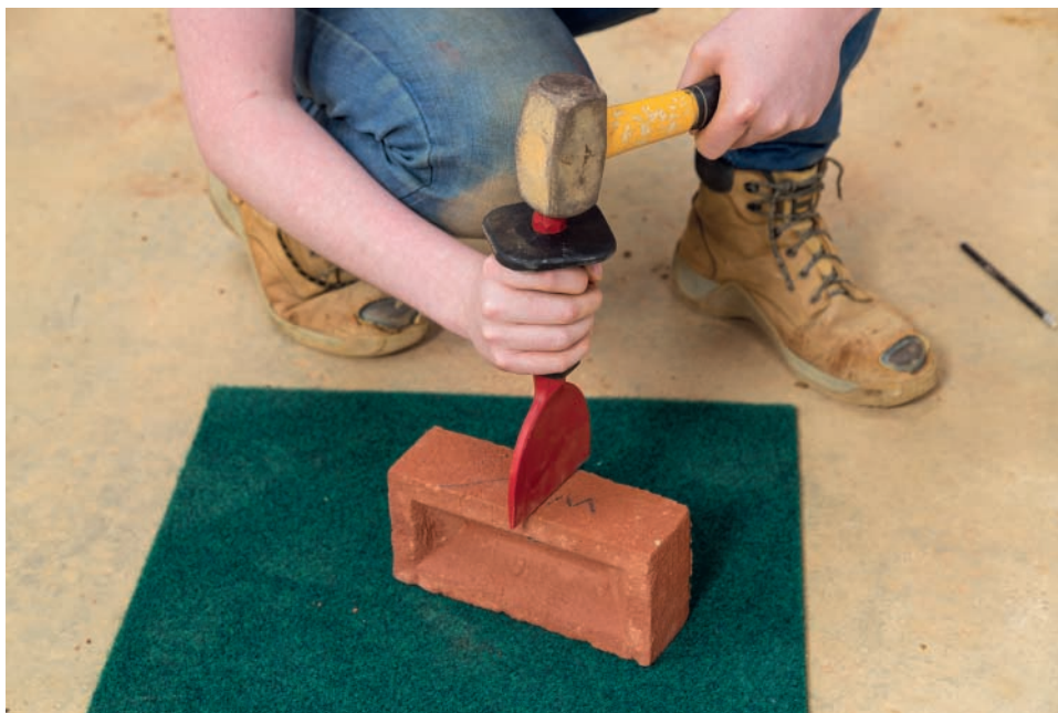
▲ Figure 4.4 Cutting a brick
