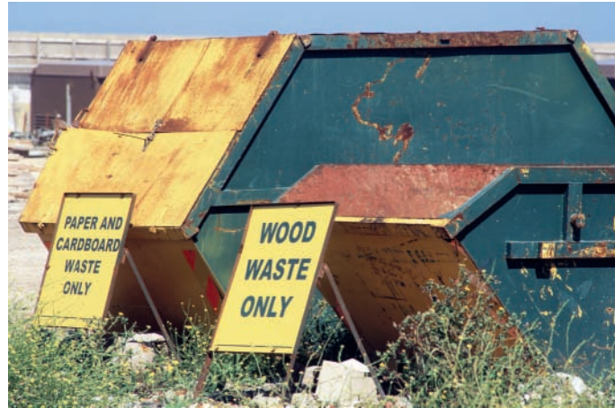
▲ Figure 1.22 Segregated waste skips on site
