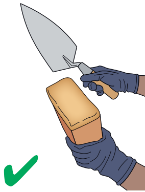
▲ Figure 4.27 Bricklayer correctly making a full perp joint
