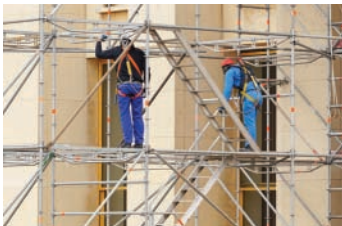
▲ Figure 6.36 Safe scaffold being set up
