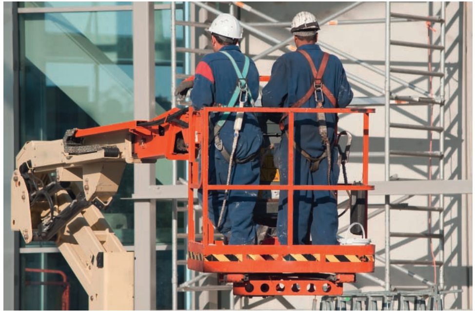
▲ Figure 6.29 Workers wearing safety harnesses on an aerial access platform
