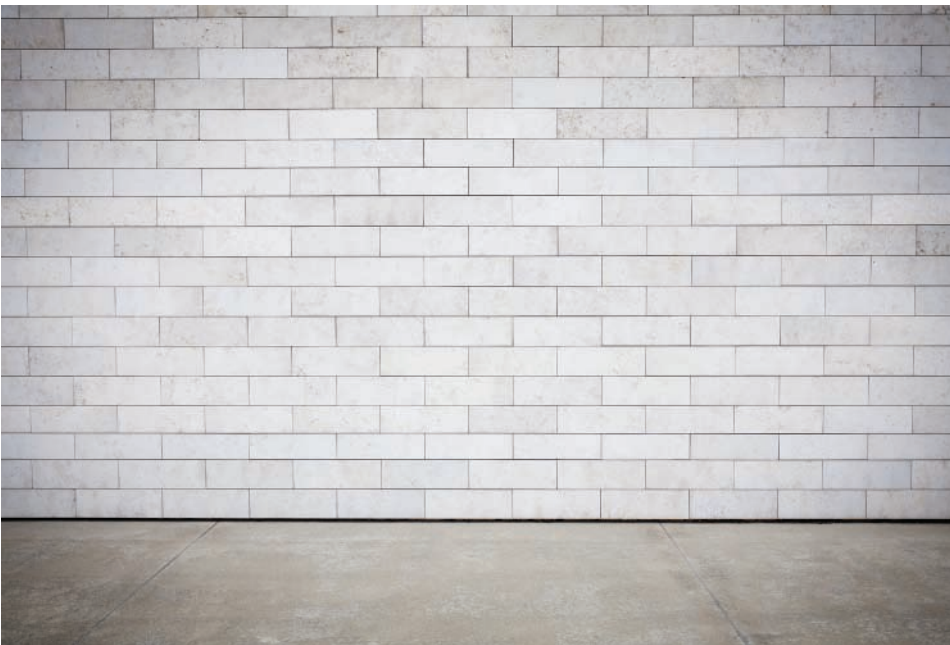
▲ Figure 5.12 A concrete brick wall
