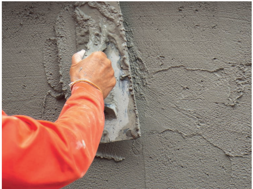
▲ Figure 1.36 Applying a coat of render to an external wall
