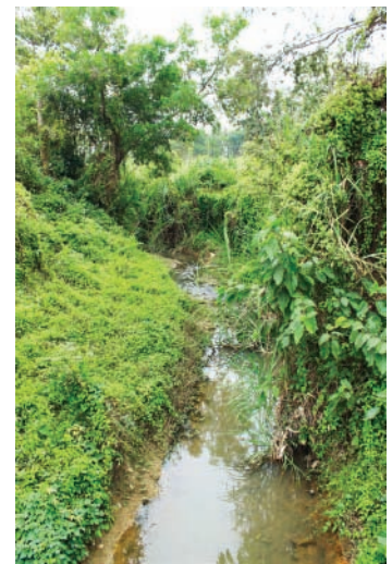
▲ Figure 2.2 Natural drainage ditches must be protected
