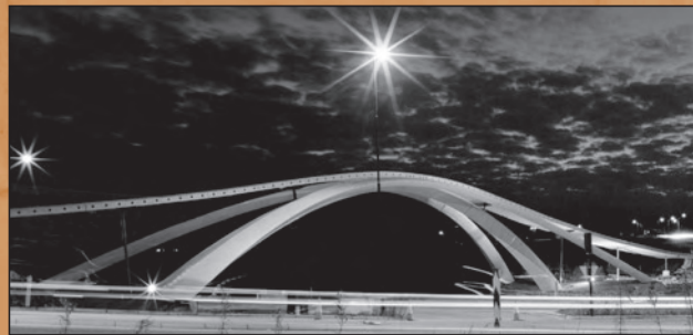
World's first Leonardo Bridge in Oslo, Norway.
