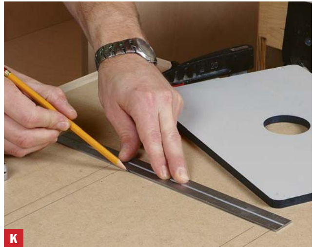
Draw the inset line Mark \frac{5}{8} " inside the first insert outline you made. You'll cut away everything inside these new lines.
