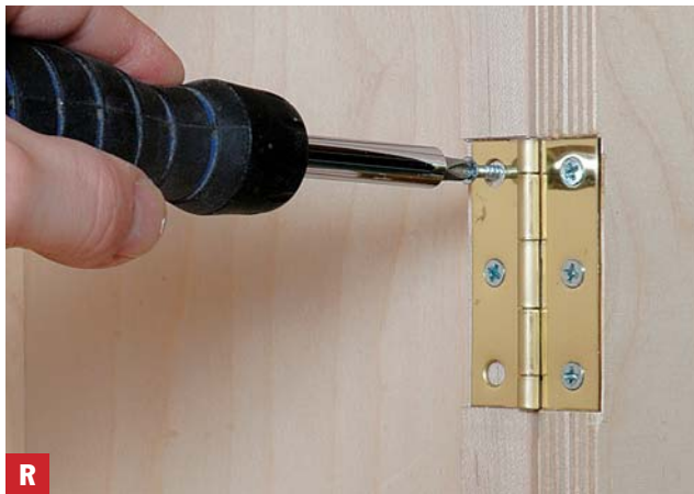
Hang the door Align the hinges into the mortises on the frame, then screw a single screw in place. If the door doesn't close flush, remove the screw and start over. Don't add additional screws until you see that the door closes flush.
