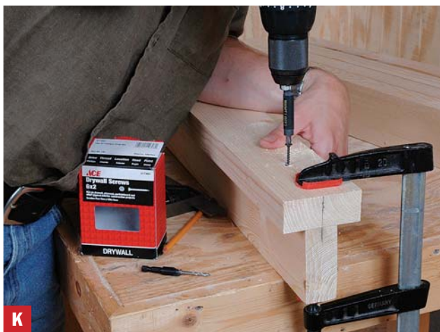
Screw the top to the subtop Be sure to drive the screws well below the surface, lessening the chance that they'll hit and damage a blade.
