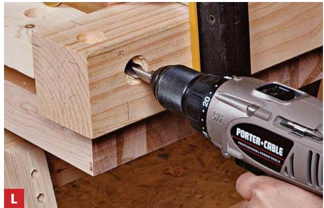
Drill for bench bolts Clamp up the front and back assembly. When the clamps are in place, use a long, ½" brad-point bit to predrill into the stretchers.
