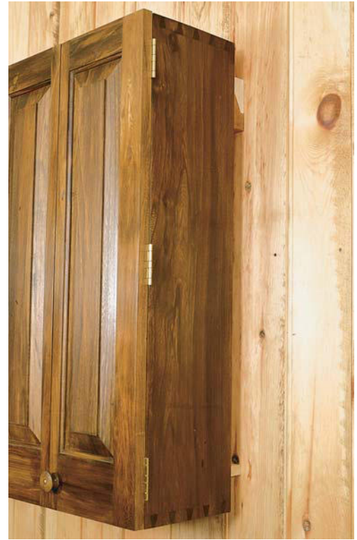
CLEATS ALLOW CABINETS TO BE MOVED. Strips ripped at 45 degrees, one screwed to the wall and one to the cabinet back, make it easy to rearrange cabinets. A kicker screwed to the cabinet back near the bottom makes the cabinet hang plumb.
