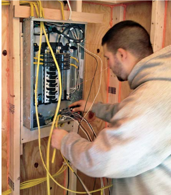
Install the wiring. St. Onge hired an electrician to ensure that all the work was done to code and that the supply was adequate for his machinery and power tools.
