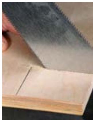
Before assembly, handsaw 3" x 3\frac{3}{4} " notches in the sides at the bottom corners to make the toe kick space.
