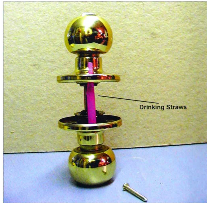
2-148. Drinking straws will help in aligning the screws when installing locksets or deadbolts on doors.
