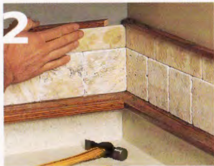
2] After the tile adhesive has dried, miter the cap pieces, and nail them in place over the top of the tile.
