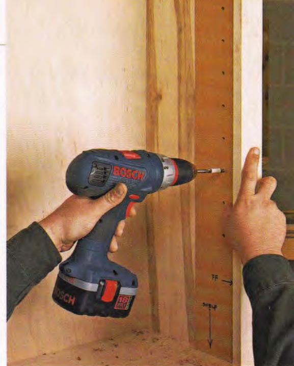
Butt the same edge of the hole template against the face frame and the divider when drilling the support holes.
