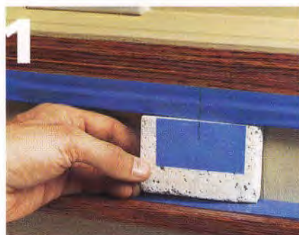
1] Align the center of the first tile with the center of the window trim. Masking tape makes the lines easier to see.
