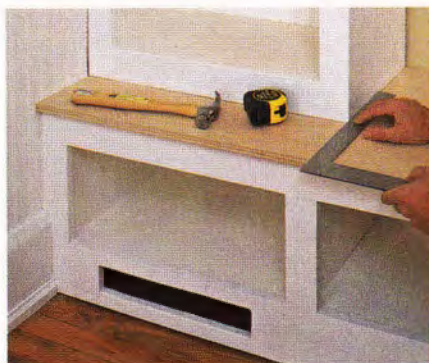
Use a framing square to make sure each tall case is positioned properly before scribing and installing it.
