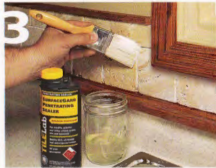
3] Porous tile and the wet conditions in the kitchen mean a couple coats of tile sealer are in order.
