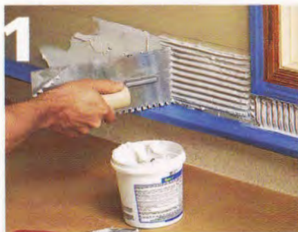
1] Use a notched trowel ( \frac{1}{4} " or \frac{3}{8} " should be fine) to spread an even bed of tile adhesive along the walls.
