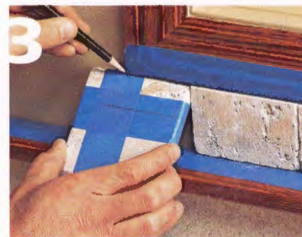
3] Now mark the tile to match the remaining space between the adjacent tile and the edge of the window trim.
