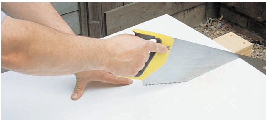
11 Cut the drawer faces to rough length.
