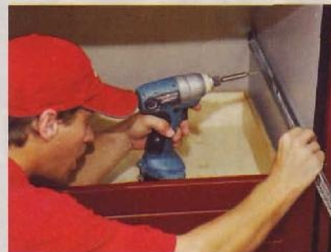
After securing and leveling the top and bottom 2"-wide steel rails, Joe McGuire fits the notched cabinet end piece against the wall (left). Once all the frames are assembled, Jake Berhow begins hanging the doors (center). Double ball-bearing drawer slides screw into factory-drilled holes (right).
