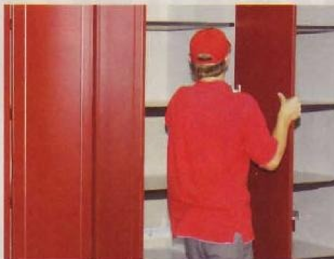
After securing and leveling the top and bottom 2"-wide steel rails, Joe McGuire fits the notched cabinet end piece against the wall (left). Once all the frames are assembled, Jake Berhow begins hanging the doors (center). Double ball-bearing drawer slides screw into factory-drilled holes (right).
