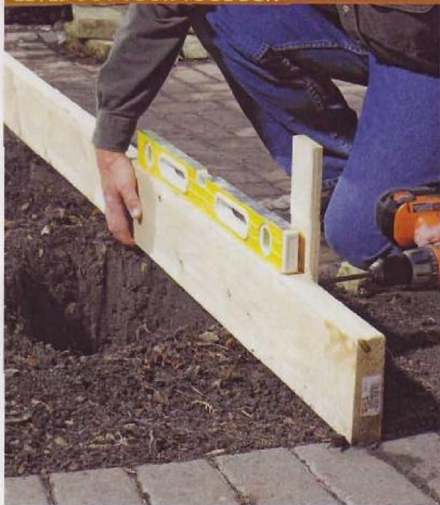
A 2' level, along with a torpedo level, is part of your basic tool kit. A 4-footer provides even better accuracy for big projects.
