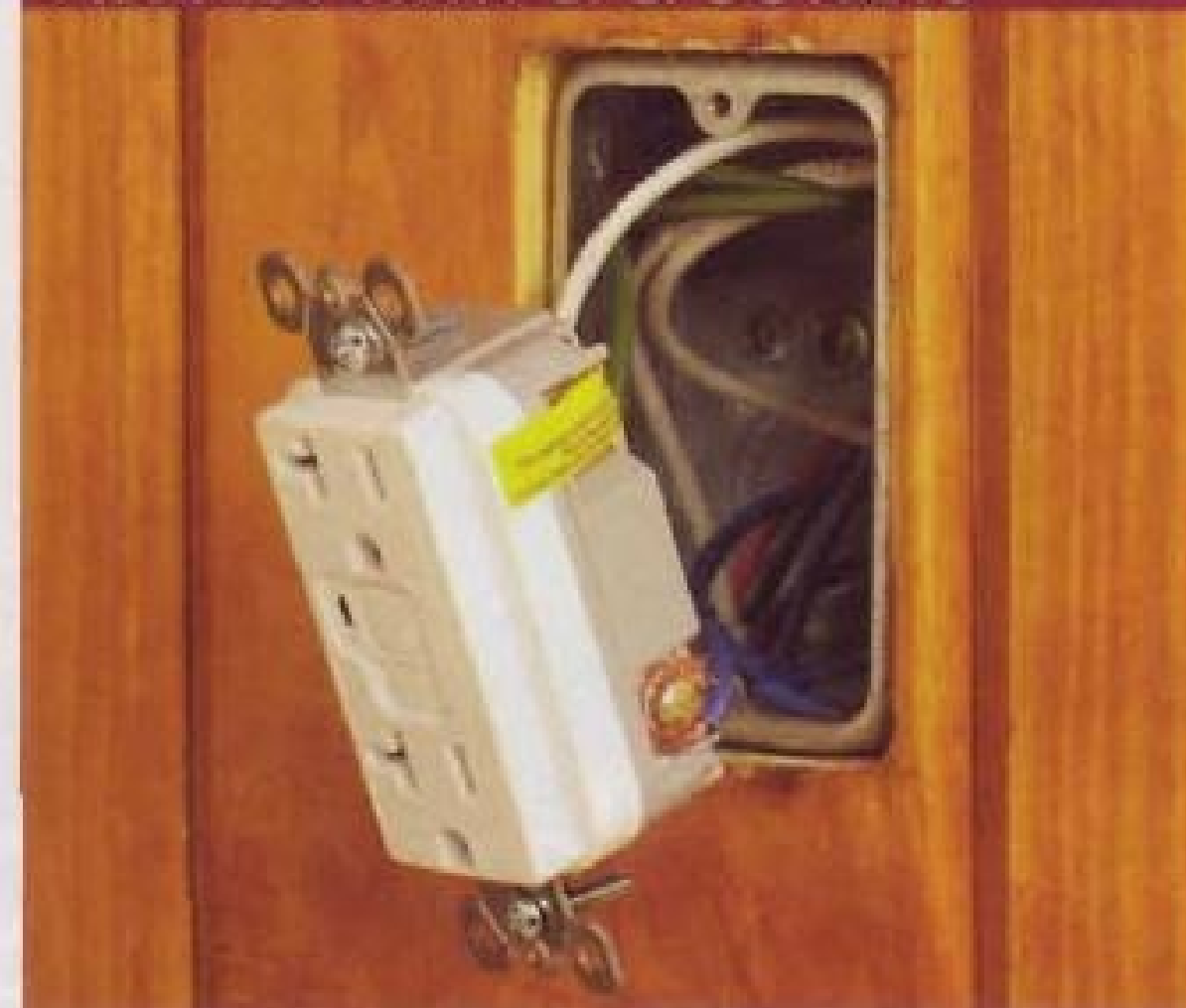
A ground-fault circuit interrupter (GFCI) duplex outlet can provide valuable protection against electrical shock.
