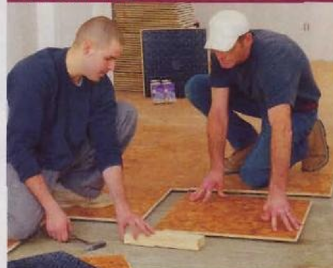
The air-gap engineered into DRlcore tiles lifts the wooden portion off the concrete, which creates an insulating layer.
