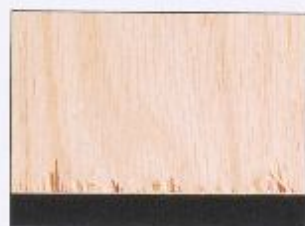
Blades on circular saws chip out fibers on the top side of the plywood.
