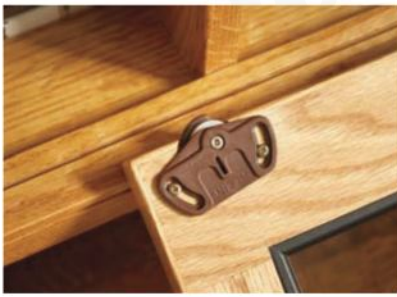
ROLLER HARDWARE allows the doors to slide easily from side to side. Moulding securing the door glass is painted black
