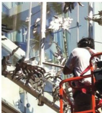
ICE BLASTING removes material quickly and requires no cleanup
