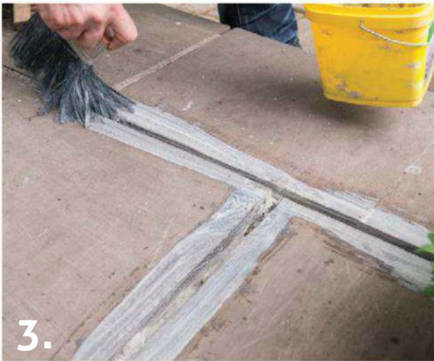
3. PAINT THE clean mortar joint with the acrylic bonding agent. This will help the new mortar bond to the edges of the stone. Don't let it dry on the top surfaces, as it will darken the stone
