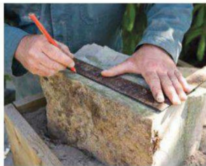
A 24" framing square is ideal for marking lines when facing a stone
