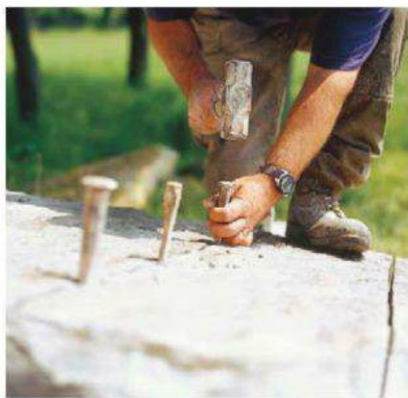
STEEL WEDGES hammered into sawn kerfs break stone along straight lines
