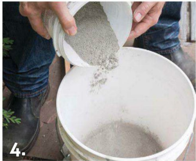
4. COMBINE THE premixed sand and mortar mix with the acrylic bonding agent. The bonding agent helps make the mortar joint more resistant to water penetration and any resulting cracks
