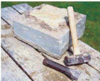
A FACED stone ready to lay on a wall. Sawn edges will be hidden within mortar joints
