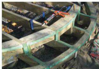
WITH THE ends of floor joists angled to match the curvature of the deck, preservative has been applied to all cut surfaces
