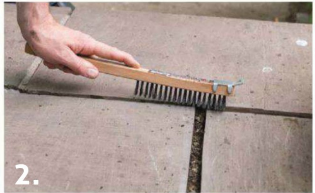
2. ONCE THE loose bits are gone, remove remaining rubble and dust with a heavy-bristled (ideally, steel) brush
