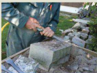
STEVE WORKS stone in a box filled with sand that sits on criss-crossed 8x8 timbers
