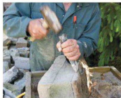
STEVE USES a 4-lb. mallet and pitching tool to face a stone
