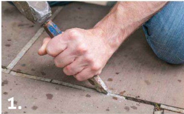
1. REMOVE LOOSE mortar by hand and clean up stubborn bits with a mallet and steel chisel
