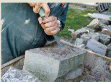
A POINT is the first tool for removing high spots on stone. Here, Steve uses a point in his largest air hammer
