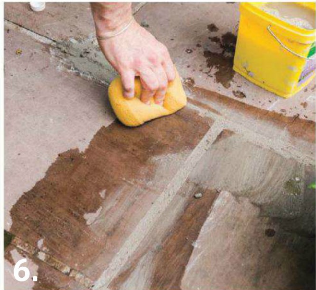
6. ALLOW THE mortar to set partially. When firm but not fully set, clean up the joint with a large, wet sponge and trowel. Remove any excess mortar from the stones surfaces to prevent staining
