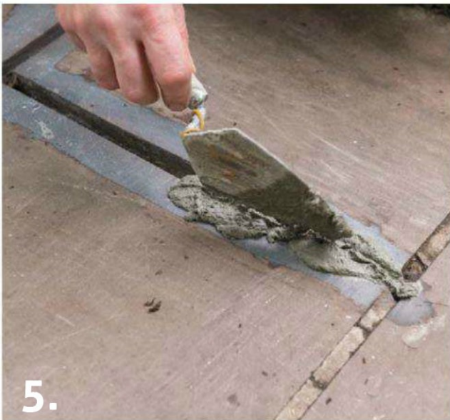
5. FILL THE joint with mortar mix, pressing it firmly into the joint with the trowel. Deep joints should be partly filled, packed, then filled the rest of the way. Remove excess mix as you work
