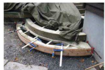
SAW CUTS partway through the rear faces of the header boards allow them to bend to the curved edge of the deck
