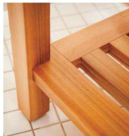
THE SHELF rests on notches cut in the lower ends of the legs
