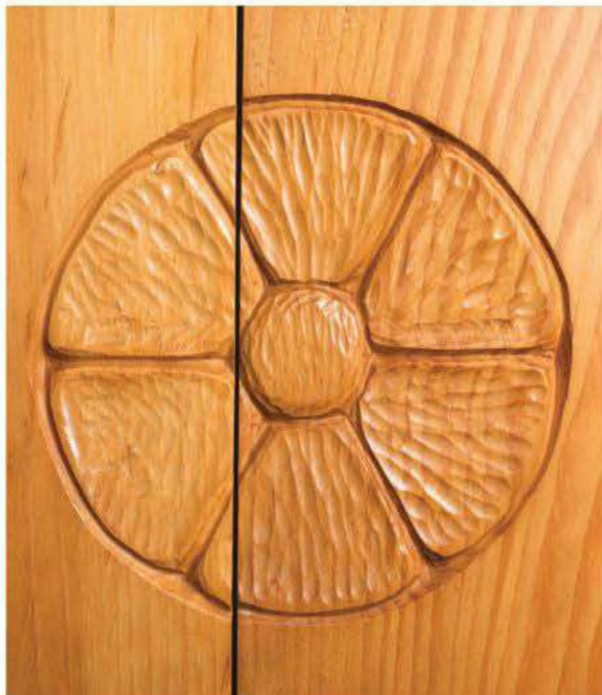
ELEVATE THE design of a simple door by breaking out the hand tools. A chisel and some time are all you need to create this elegant detail
