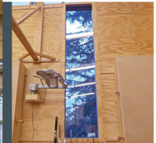
Frank installed double-pane insulated glass in 24x96" frames he built in his shop from 2x6 fir and cedar trim.
