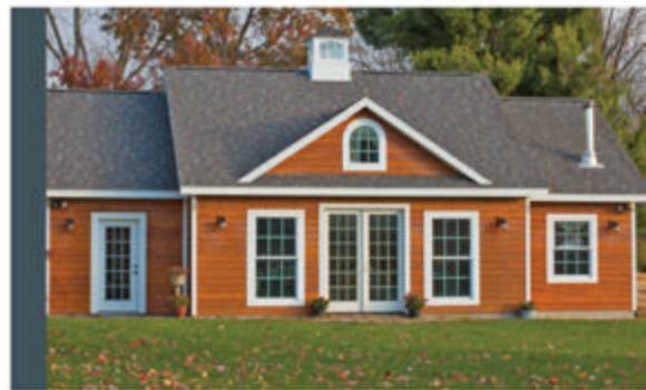
Ruth modified the footprint of a four-car garage. She added a bump-out and large windows, and topped it off with a cupola she designed and built.
